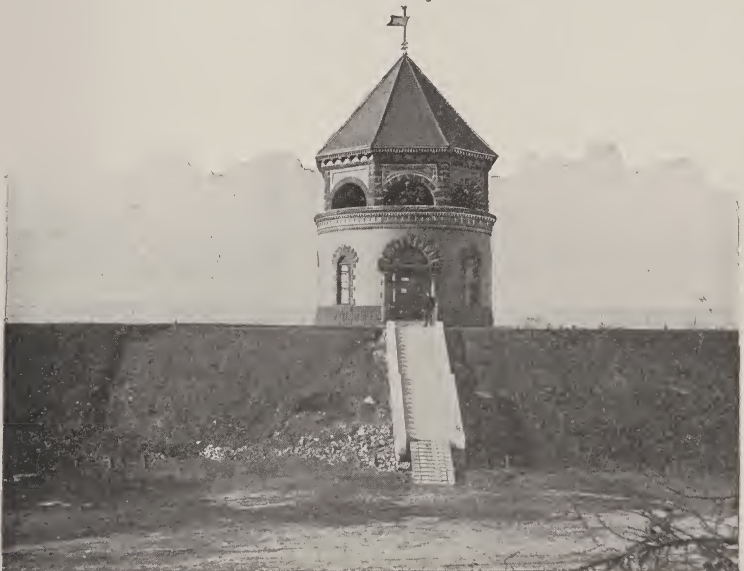
FIG. 85.—PAYSON PARK GATE-HOUSE, CAMBRIDGE.
