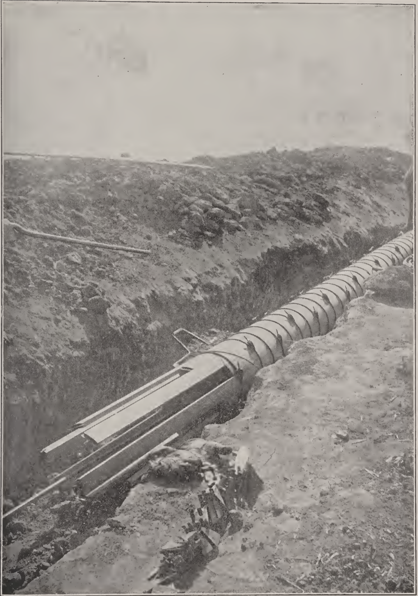
FIG. 147.—WOODEN-STAVE PIPE.
