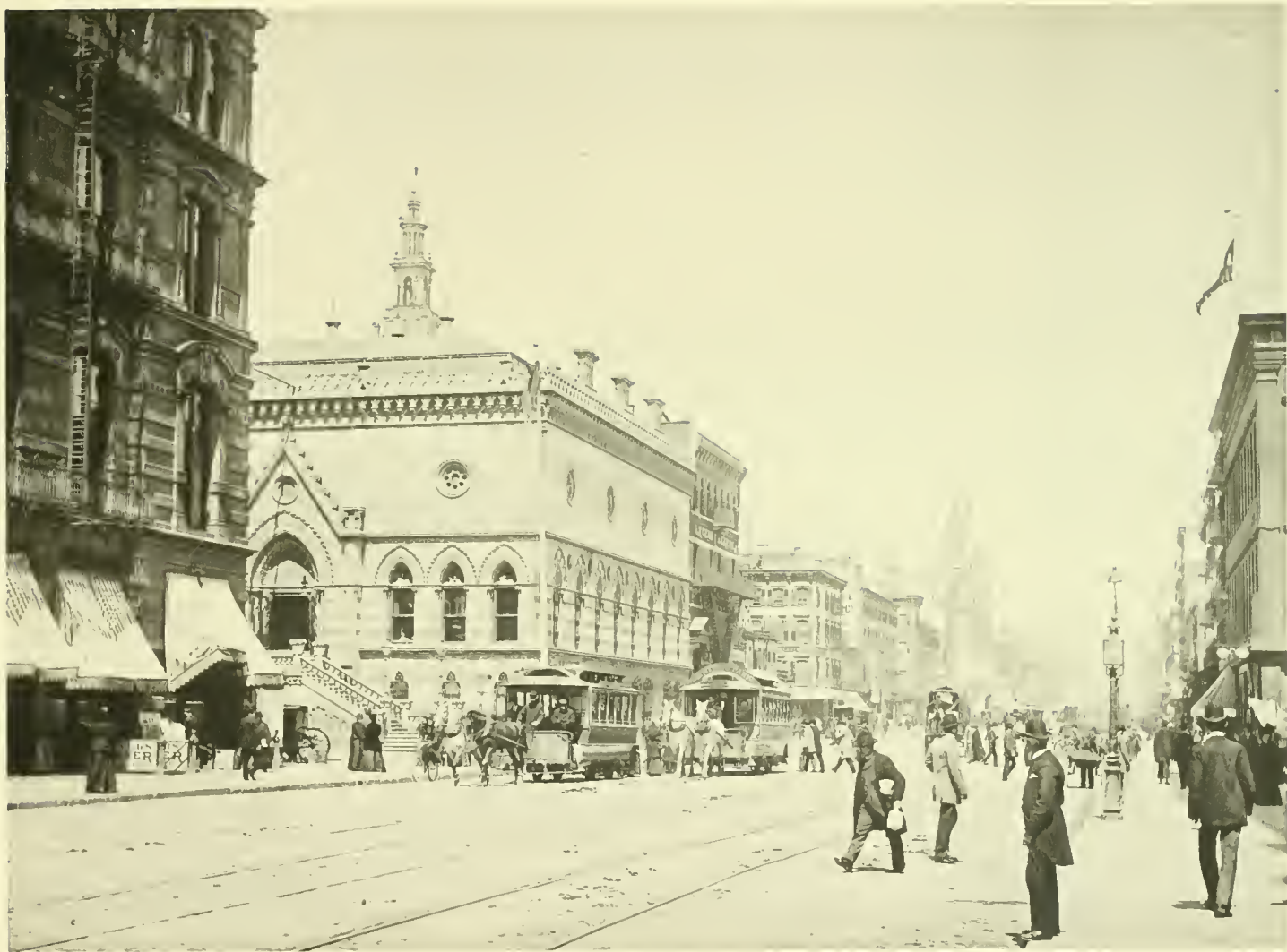
ACADEMY OF DESIGN AND FOURTH AVENUE ABOVE 23rd STREET
