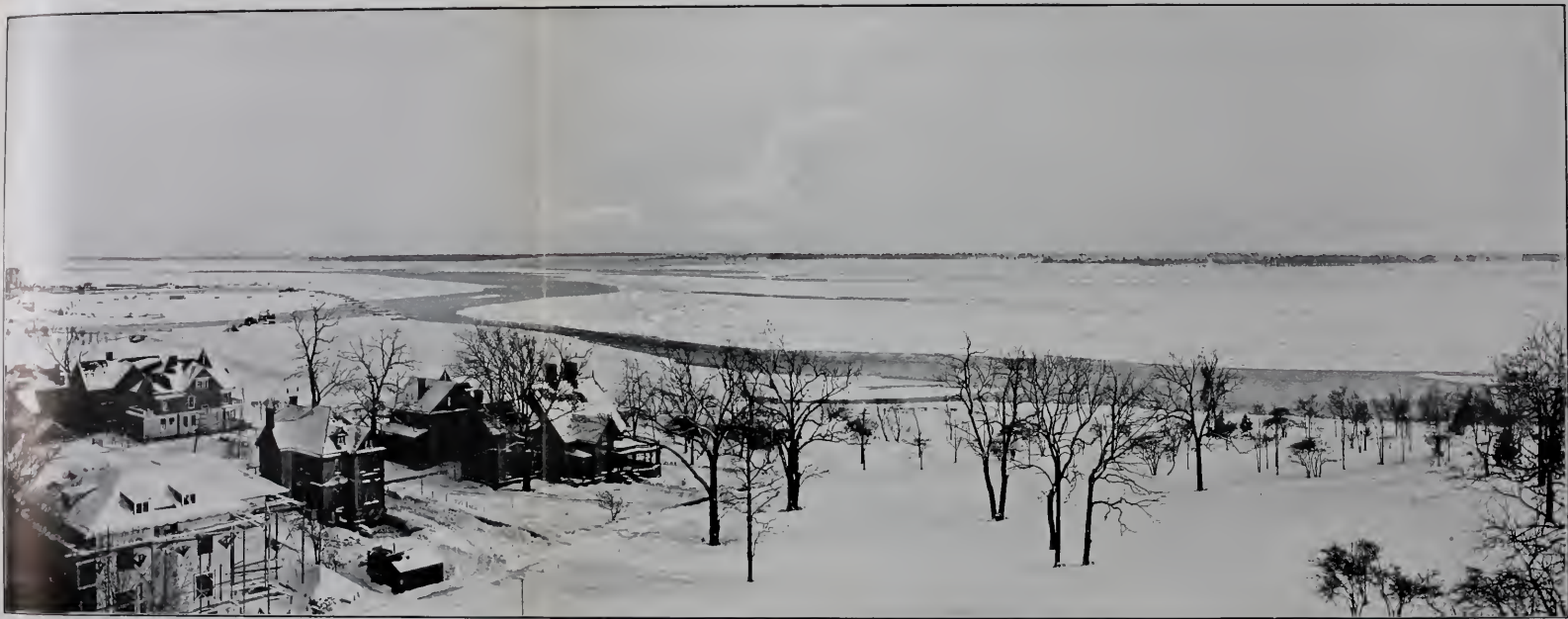
FIGURE No. 557-S - Showing during the winter of 1905 small channels created by blasting and breaking up the ice by means of dynamite, to secure water at the intake of the Niagara Falls Hydraulic Power and Manufacturing Co.
