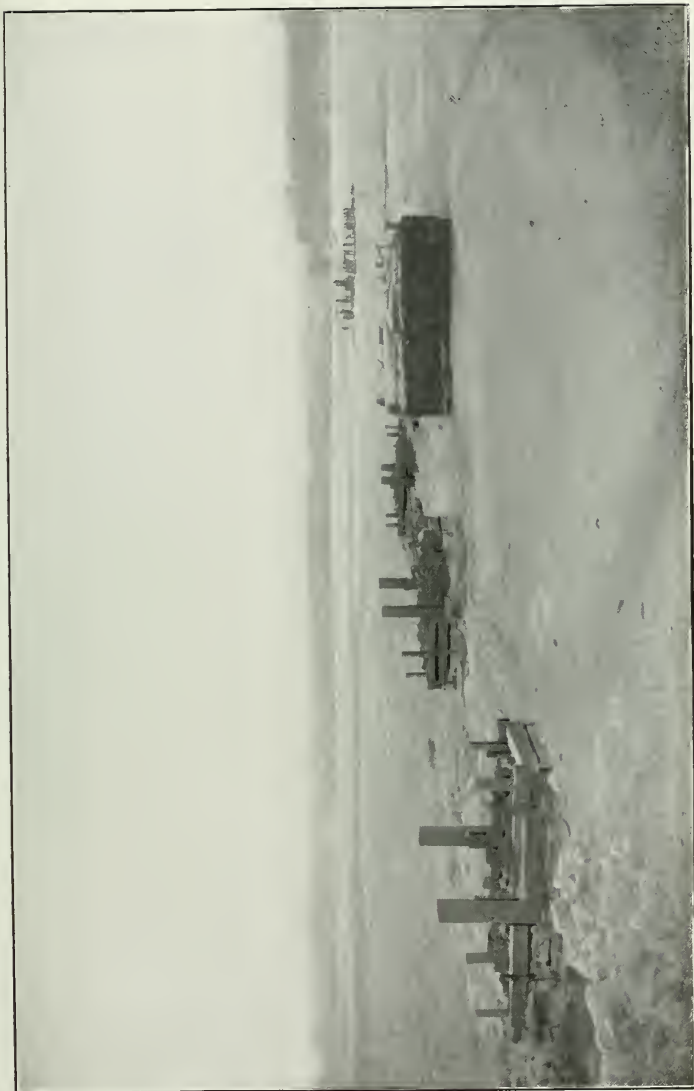
PHOTO No. 1434c.—Showing Ice Fields obstructing the Intake of the Niagara Falls Power Co. Putting in cribs and booms at the mouth of the Canal for protection against ice.
