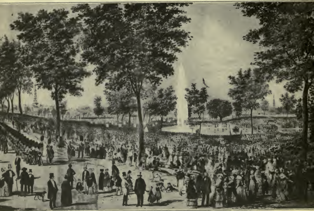
THE FUSILIERS (BAT. F, 55TH), ON COMMON AT INAUGURATION OF COCHITUATE WATER SYSTEM, OCT. 25, 1848
