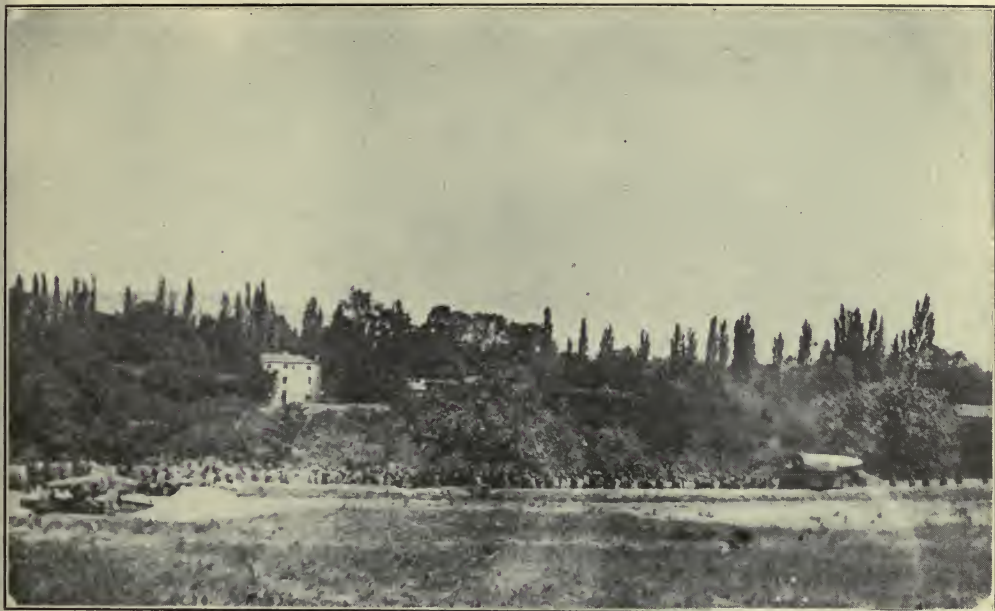
BATTERY IN POSITION
