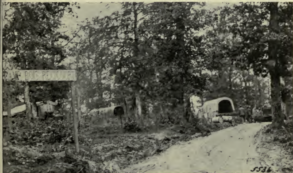
NEAR P. C. SEVIER, ENTRANCE TO REST-CAMP
