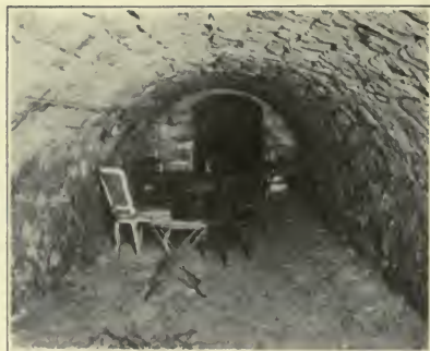
Signal Corps Photo WINE-CELLAR USED AS P. C.
