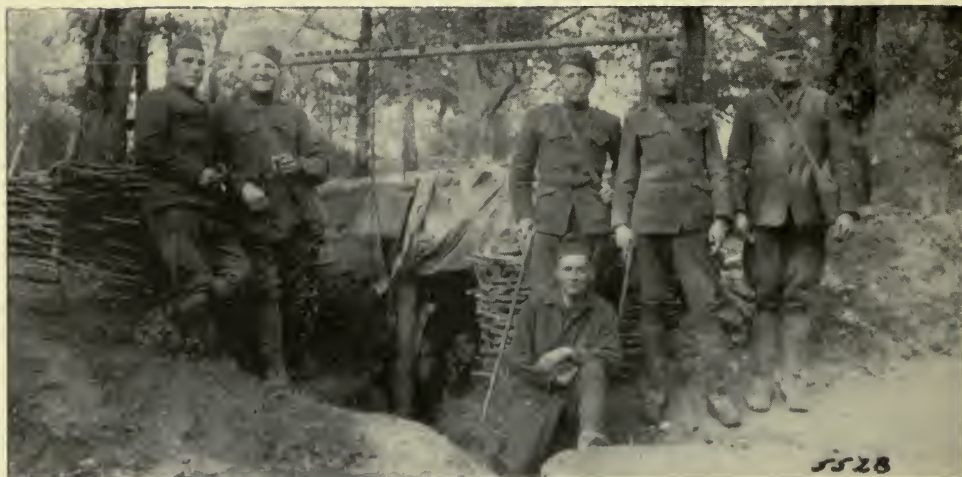
REGIMENTAL TELEPHONE CENTRAL IN THE BOIS DE RECICOURT
