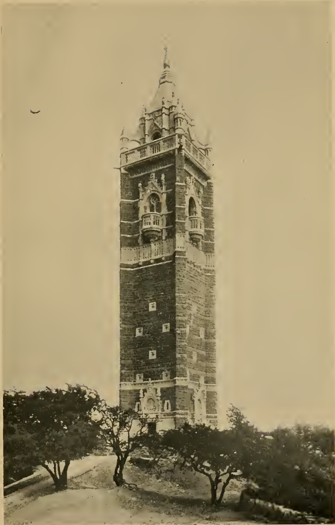
THE CABOT TOWER, BRISTOL, ENGLAND.
