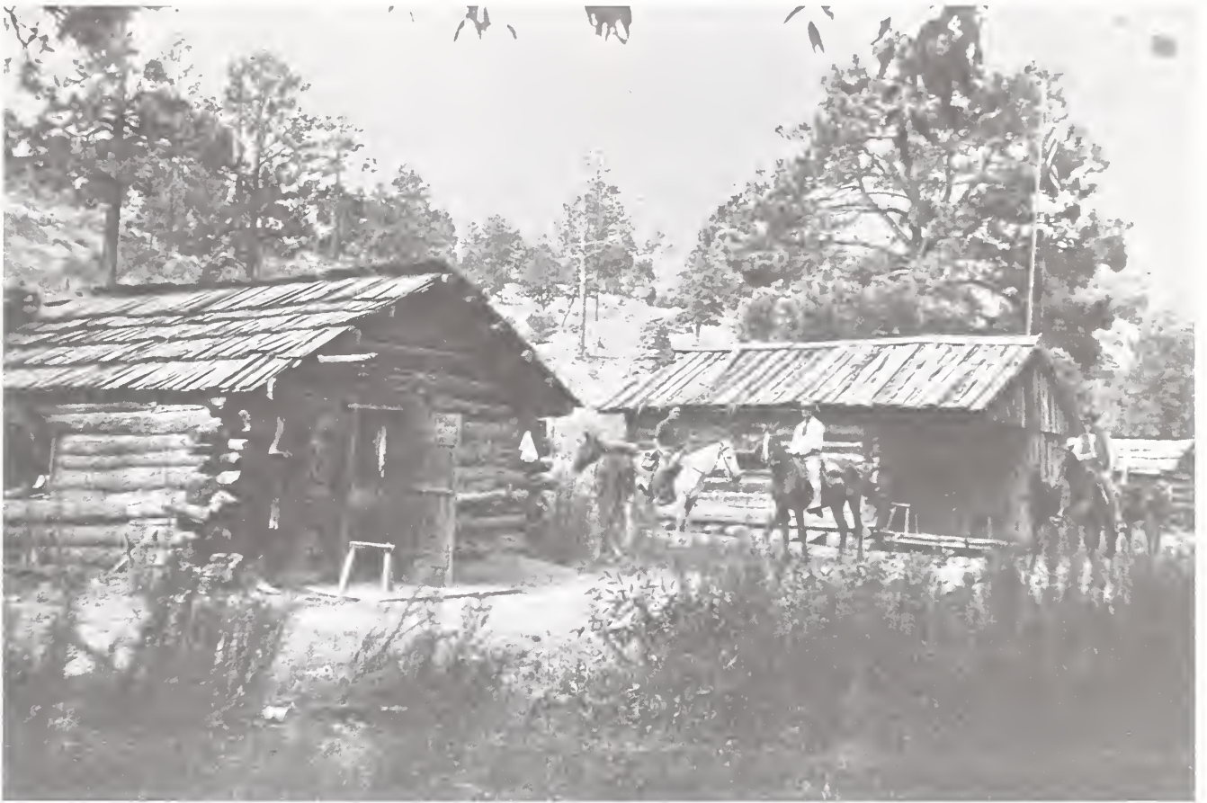
Figure 4. Old Bear Canyon Ranger Station, Gila National Forest, in 1907. This was not a Forest Service constructed layout but one which in the run of places in those days was found and occupied by Forest officers in lieu of anything else. A Geological Survey crew was camped at the station and the two horses at left belong to that outfit. A Geological Survey man is on the white horse. Ranger Andrews is on the horse at right.; the man on the black horse is Douglas Rodman, at that time Forest Supervisor.
