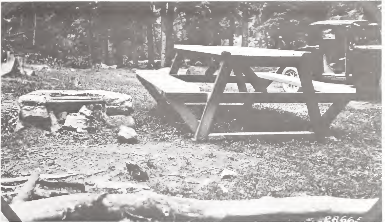
Figure 22. Table and fireplace at Rio Gallinas Campground, Santa Fe National Forest. Built by the Rio Gallinas Civilian Conservation Corp Camp. Photo by John D. Jones, October 1933.
