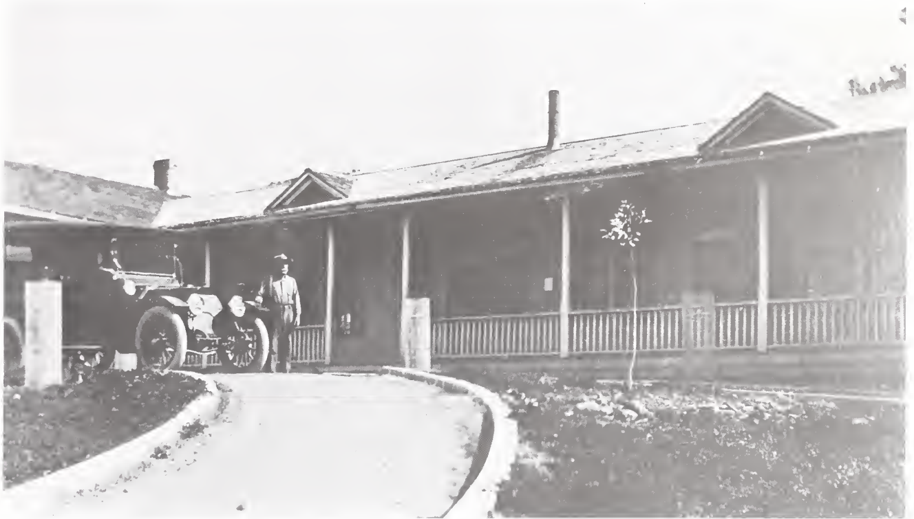
Figure 6. Tonto Supervisor's Cottage at Roosevelt, Gila County, Arizona, May 27, 1913.
