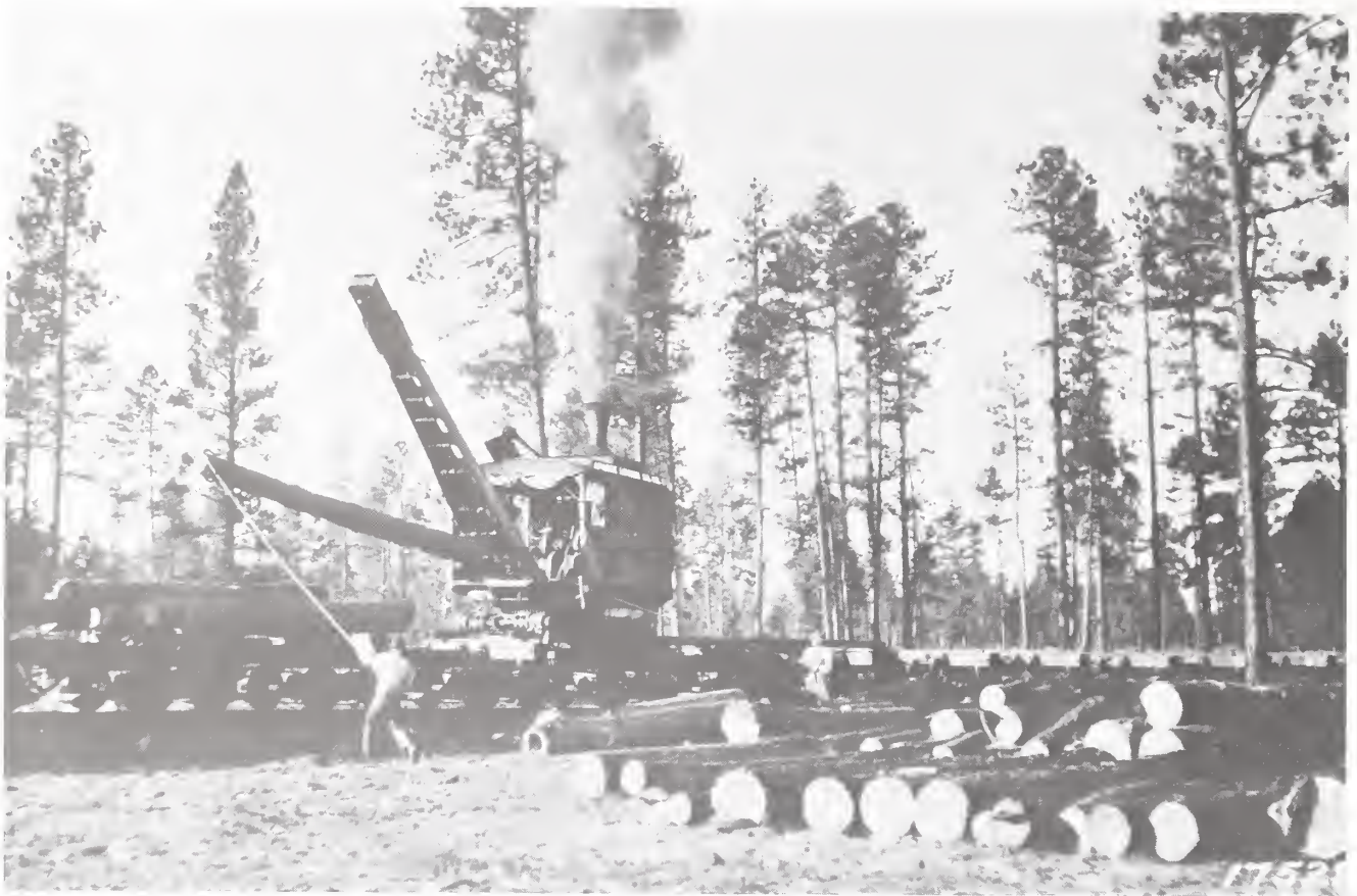
Figure 34. A steam loader, mounted on a railway car, easily handles logs on this Apache Lumber Company Sale. Photo by Paul H. Roberts, 1902.
