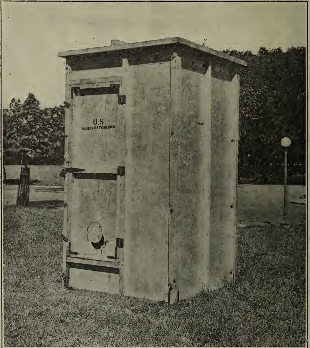
Smokehouse, as described, door and top closed, draft port partly open.
