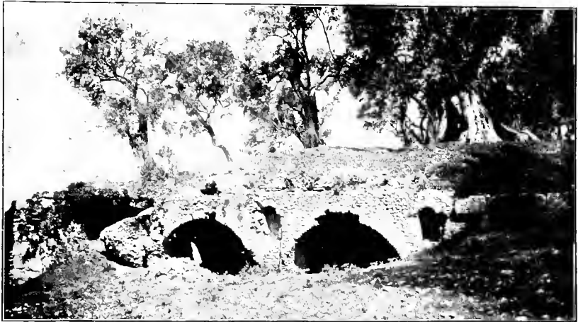
Sand and Pebble Catch-tanks near Tivoli. Dimension-stone aqueducts of Marcia at either end of the tank built of small stone; opus incertum . The arches are chambers of the tanks.
