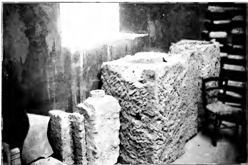
Roman water-pipe made of bored-out blocks of stone.
