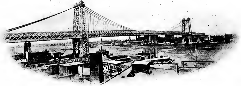
FIG. 43.—New East River Bridge.
