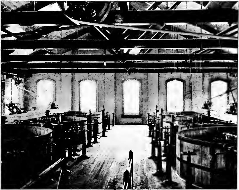
The Jewell Filter-plant at Norristown, Penn.
