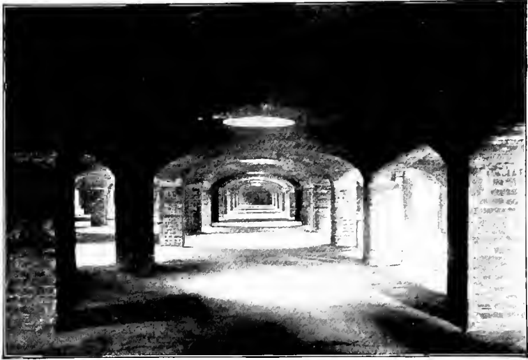
Interior of Covered Filter at Ashland, Wis.
