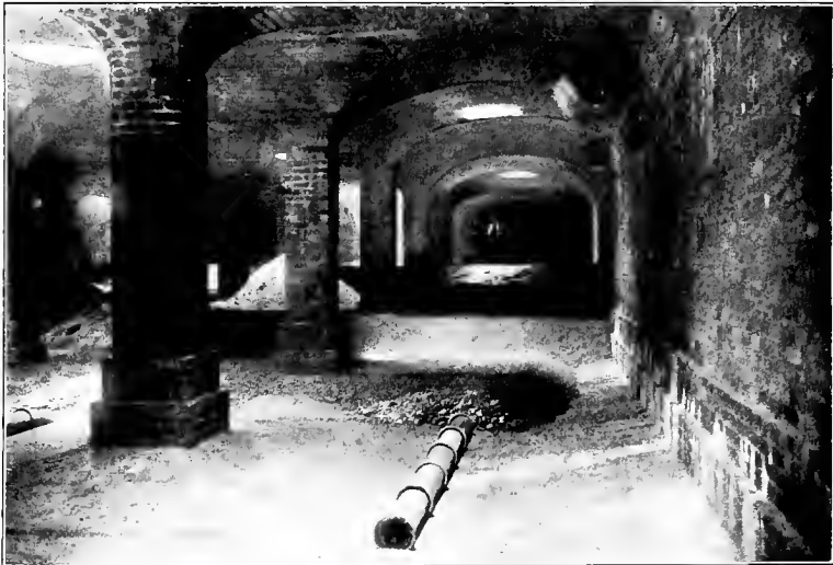
Partially Filled Covered Sand Filter showing Drain pipe.
