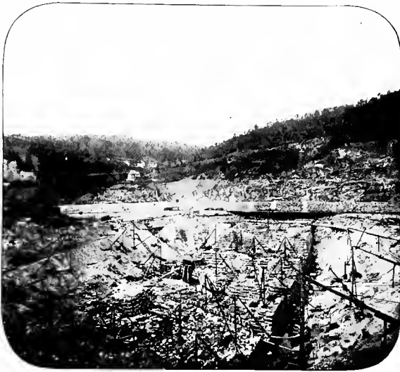
Foundation Masonry of New Croton Dam.
