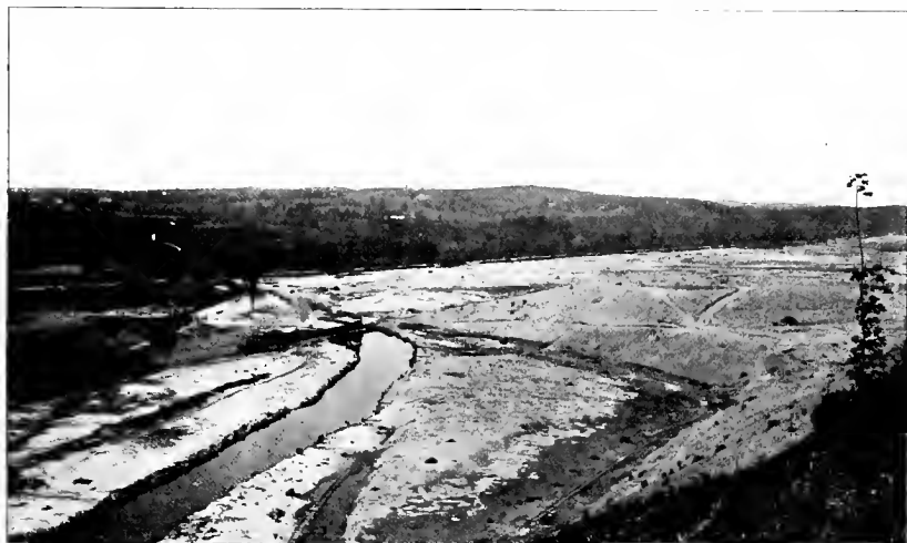
Wachusett Reservoir, showing Stripping of Soil.
