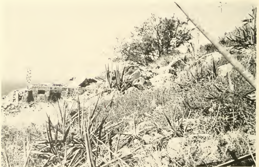
2. The upper level, Redonda. Former "residence" of phosphate-mining crew at left; rain-water cistern at extreme right.
