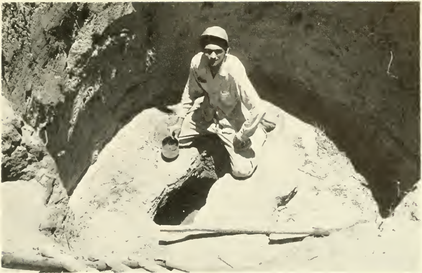
1. A shallow dug well reaches the water table below the dunes and supplies drinking water for a household during the long drought.
