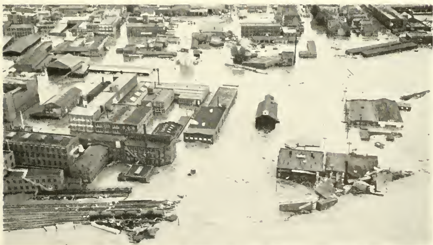
2. Flood damage due to invasion of flood plain by industry. Photograph courtesy of Sikorsky Co.
