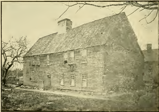
Saltonstall House, Ipswich
