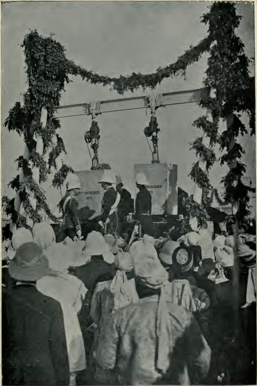
HIS MAJESTY LAYING THE FOUNDATION STONE OF NEW DELHI
