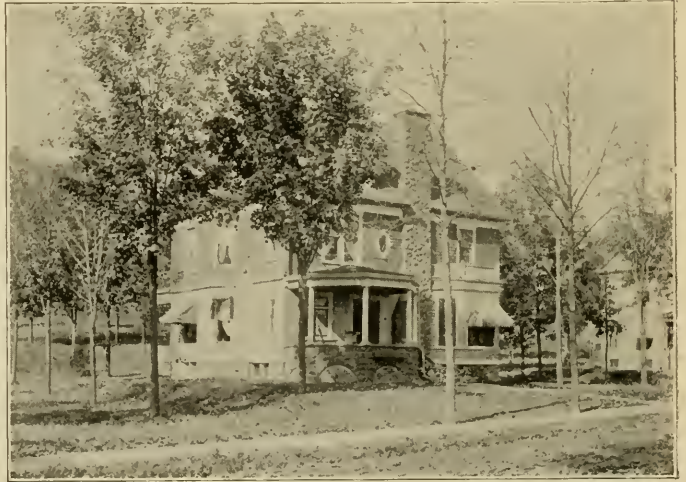
P. R. YOUNG'S RESIDENCE, WEST STREET.
