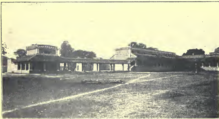
NEW WING AT LUCKNOW HOSPITAL.
