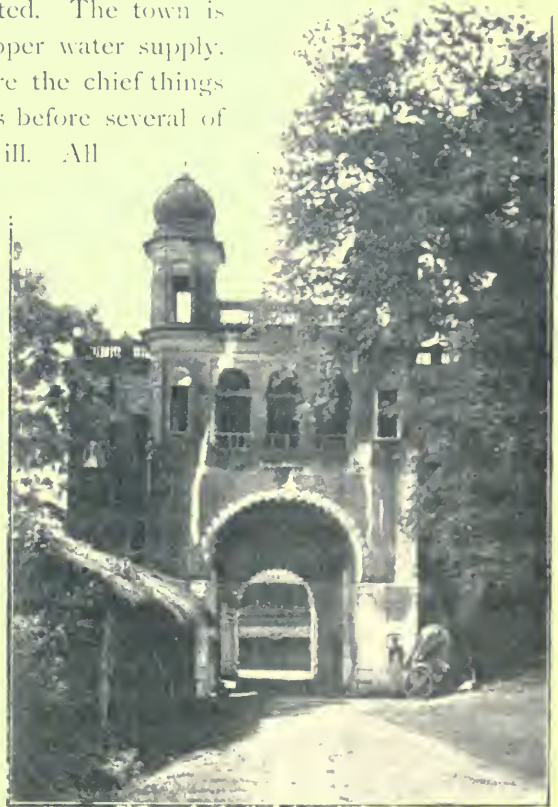
OLD GATEWAY AT PATNA. Entrance to Hospital Grounds.
