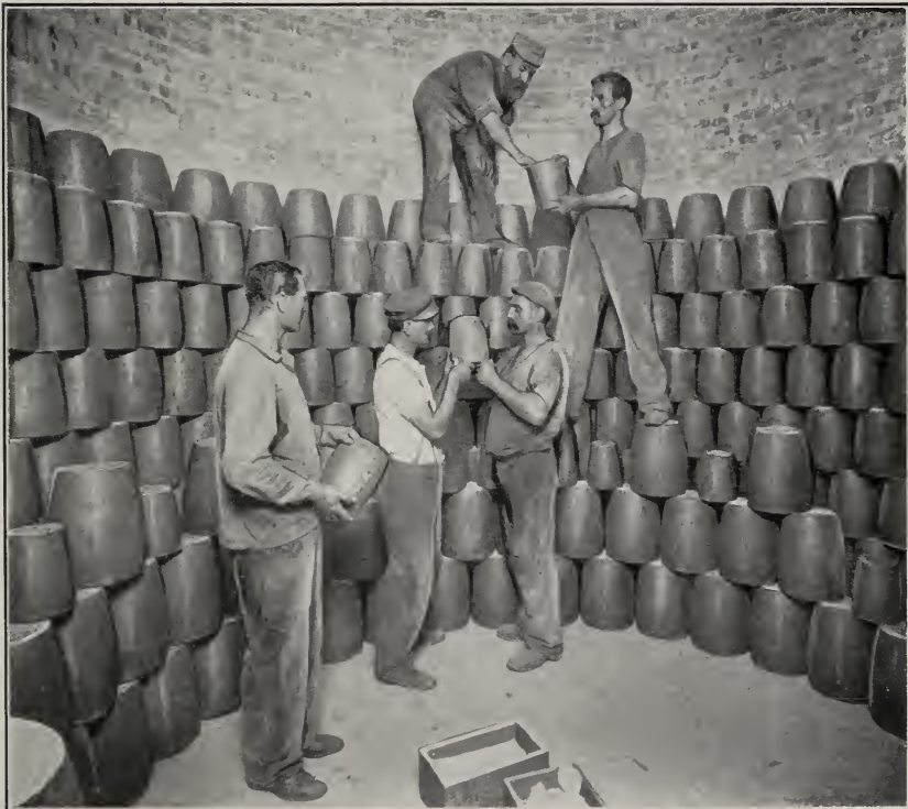
SCENE IN THE DIXON FACTORY—INTERIOR OF A KILN
