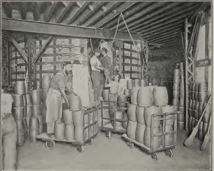
SCENE IN THE DIXON FACTORY—LOADING UP A KILN
