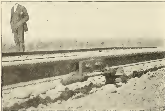
Third Rail Disconnecting Switch.
