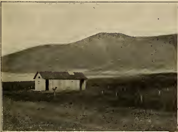
Pumping Plant at Young Grove, at Exeter.
