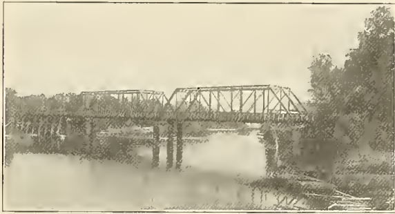
Steel Bridge Over the Feather River at Marysville.
