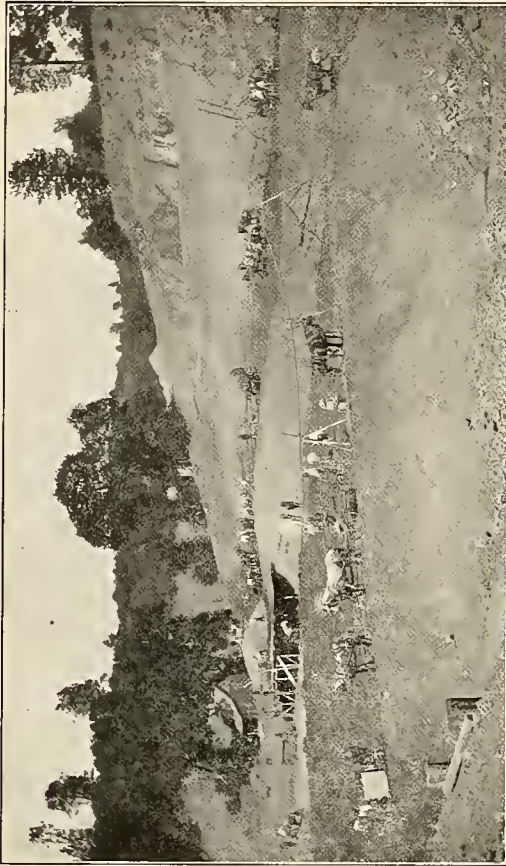
Lake Arthur Dam During Construction.
