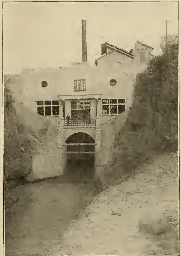
Hydro-electric Plant of Holtville Power Company.
