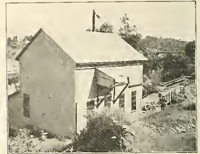
Secondary Plant at Folsom Power Station. Run by Outflow from First.
