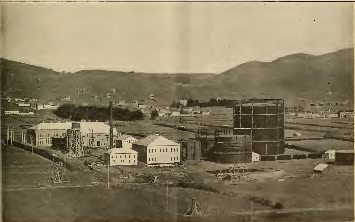
General View of Martin Station at Visitation Valley, near San Francisco—The First Large Producer of Oil-Gas in the World.
