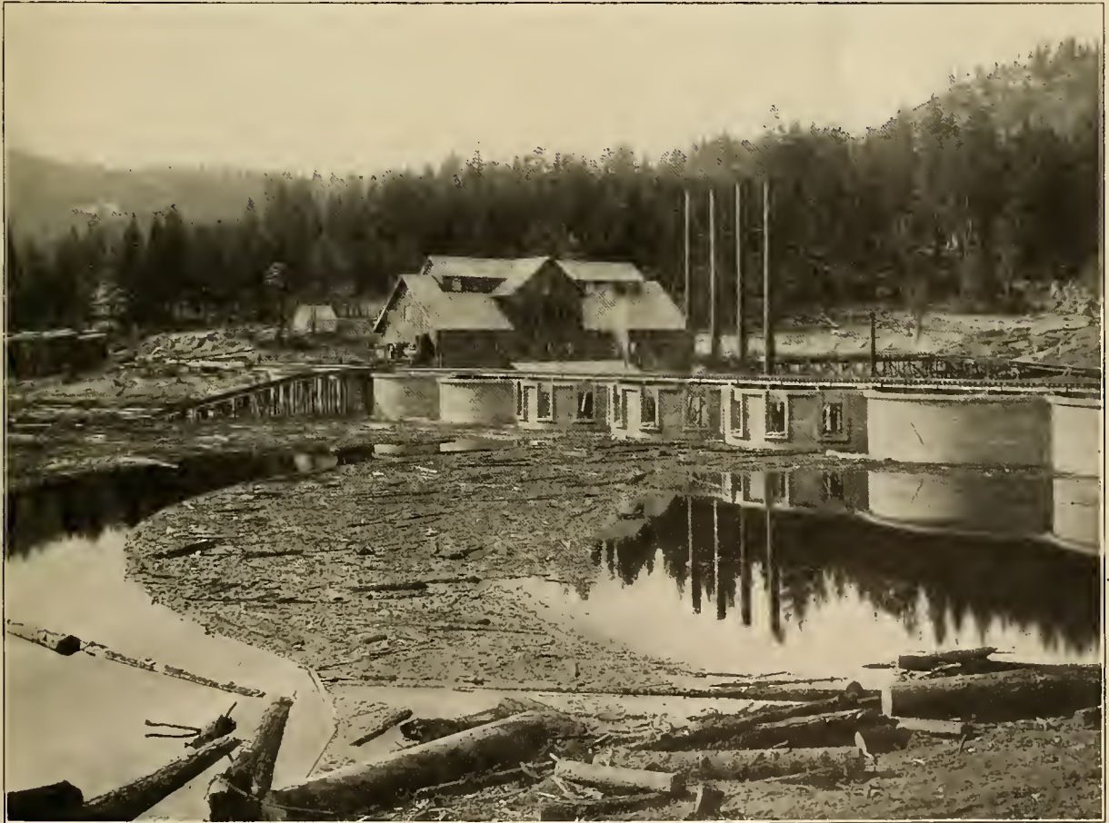
Completed Multiple Arch Dam at Hume, California.
