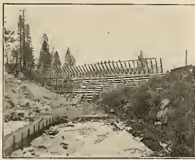
Constructing the Lake Vera Dam in 1898
