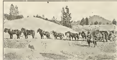
Hauling Machinery to Power House in 1865
