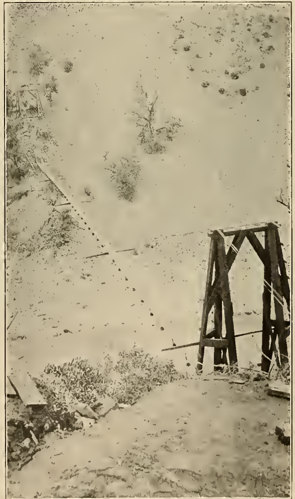
Suspension-foot-bridge below Dam-site to Administration Quarters.
