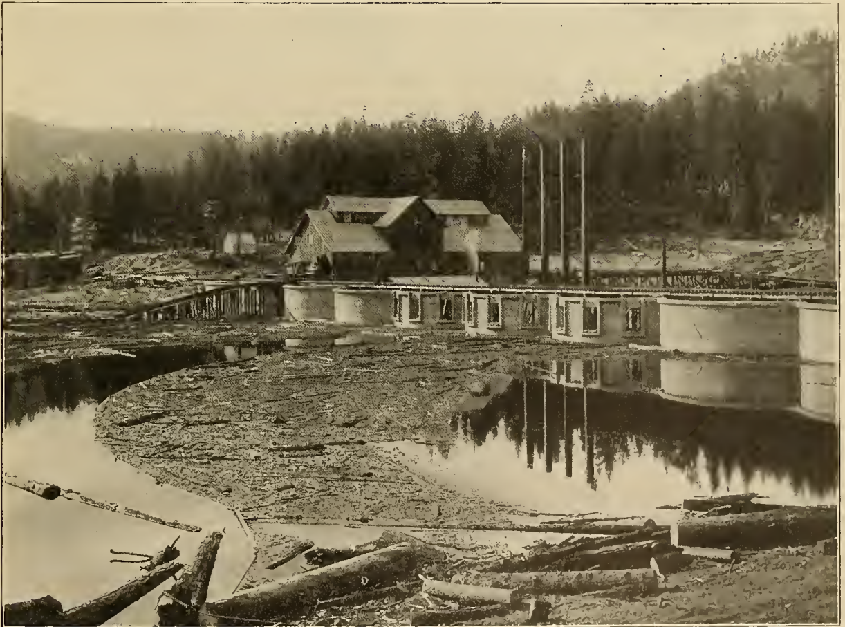
Multiple Arch Dam at Hume, California.
