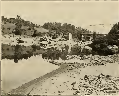
County Bridge Across American River, also Old Stone Abutment that supported first Transcontinental Railroad Bridge.
