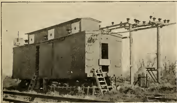
Portable Transformer Station.
