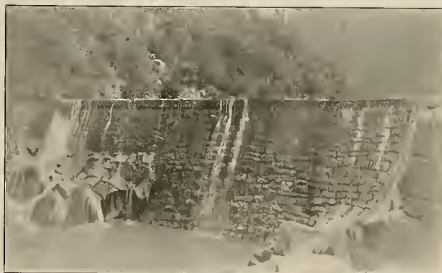
The River Dam as It Looks To-Day With Its Heavy Facing of Granite,
