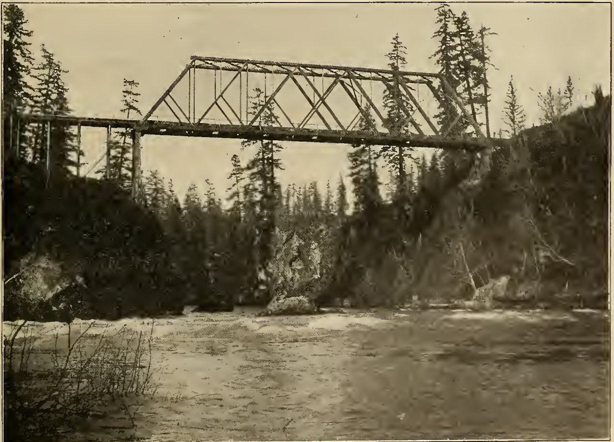
Site for 80-ft. Dam at Mill Bridge, near Estacada.
