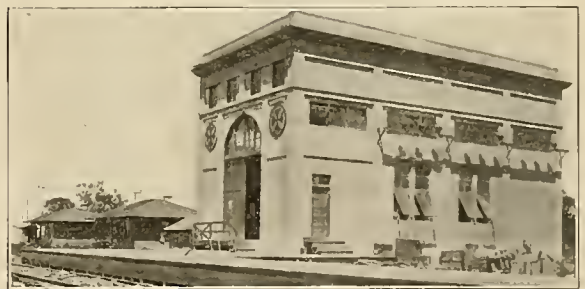
Sub-Station No. 8 at Nicolaus.
