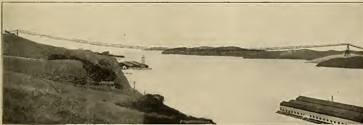
The 4427 ft. Span of the Pacific Gas & Electric Co. Across Carquinez Straits.
