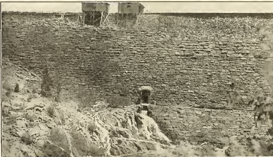
Downstream Face of Fordyce Dam.
