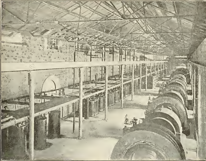
Interior View of Colgate Power House.
