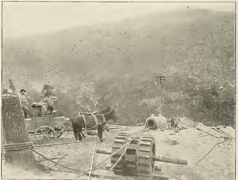
Where the Massive Machinery was Unloaded at the Top of the Ridge to be Skidded Down half a Mile.
