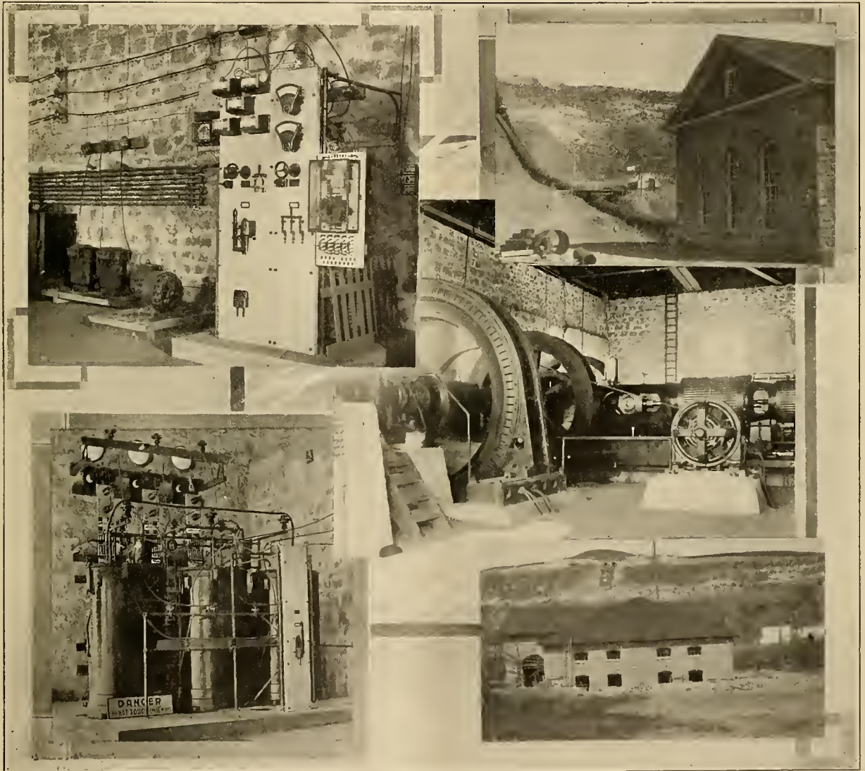
Plant of Yakima-Pasco Power Co. at Naches, Wash.
