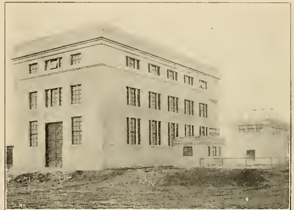
Sub-station at Brighton, showing Sectionalizing-house in background; Pumphouse and Cooling Tank in right foreground.
