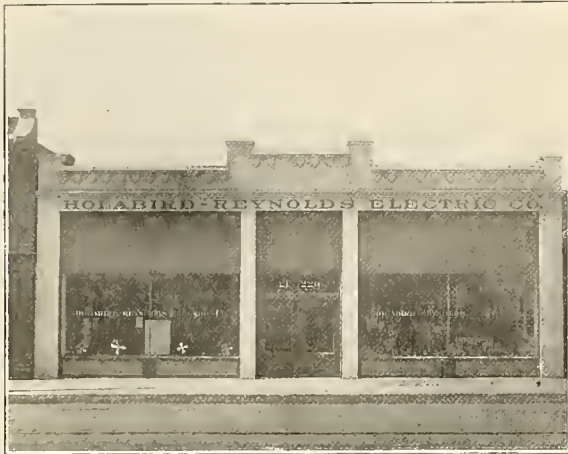
Exterior of Los Angeles Store.
