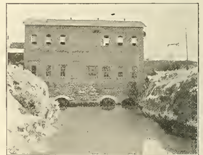
Folsom Power House, with Outflow Canal Through Solid Granite.
