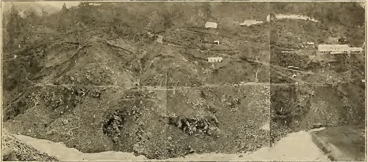
South Bank of the Feather River at the Intake. Crib-dam in the Right Foreground; Compressor-house and Cook-house on the Right; Stables and Camp in the Right Background; Transformer-house in Center Background; South End of Proposed High Dam in Center Foreground; Quarry in the Left Foreground; Keystone Drill in the Left of Picture.
