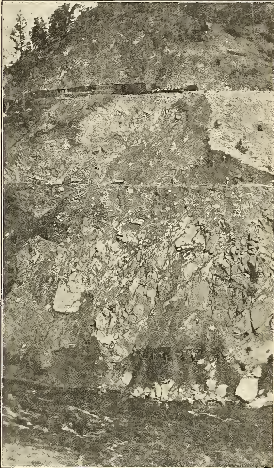
North End Site of Proposed High Dam. The Crest will Reach to a Point about half-way between the Railroad-track and the Road on which the Dump-carts can be Seen. A Test-hole can be Seen in the Upper-right Side of the Picture.
