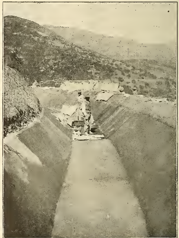
Section of Concrete Ditch for Tule Plant
