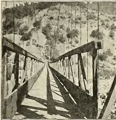
Suspension Bridge across Yuba River at Colgate
