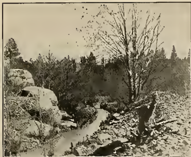
The Ditch Flowing into Lake Vera bringing Water from the Deer Creek Power House
