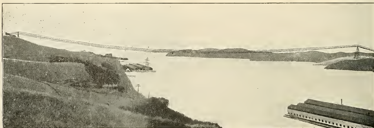
The 4427 ft. Span of the Pacific Gas & Electric Co. Across Carquinez Straits.
