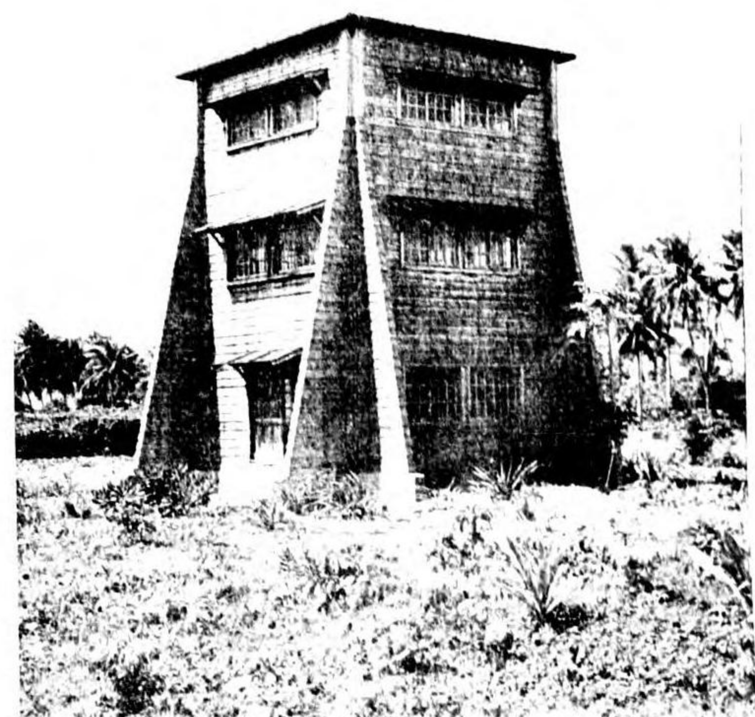
HIGH FREQUENCY TOWER (OPERATOR AND RECEIVER ARE ON SECOND FLOOR)
