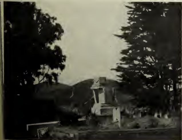
A DAMAGED MONUMENT IN LAUREL HILL CEMETERY, SAN FRANCISCO.
