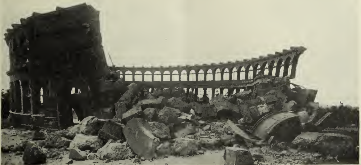
THE PANORAMA, A CONCRETE STRUCTURE WRECKED BY THE EARTHQUAKE Golden Gate Park, San Francisco
