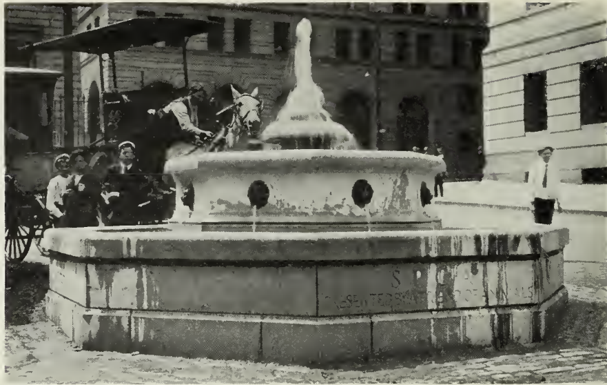
GRANITE DRINKING FOUNTAIN, BALTIMORE. Wyatt & Nolting, Archts.
