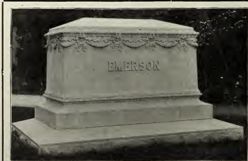
Emerson Monument, Spring Grove Cemetery, Cincinnati, Erected by the Harrison Granite Company
