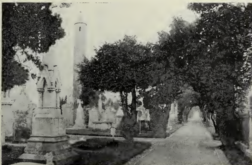
LOOKING EAST, INSIDE THE OLD ENTRANCE T
