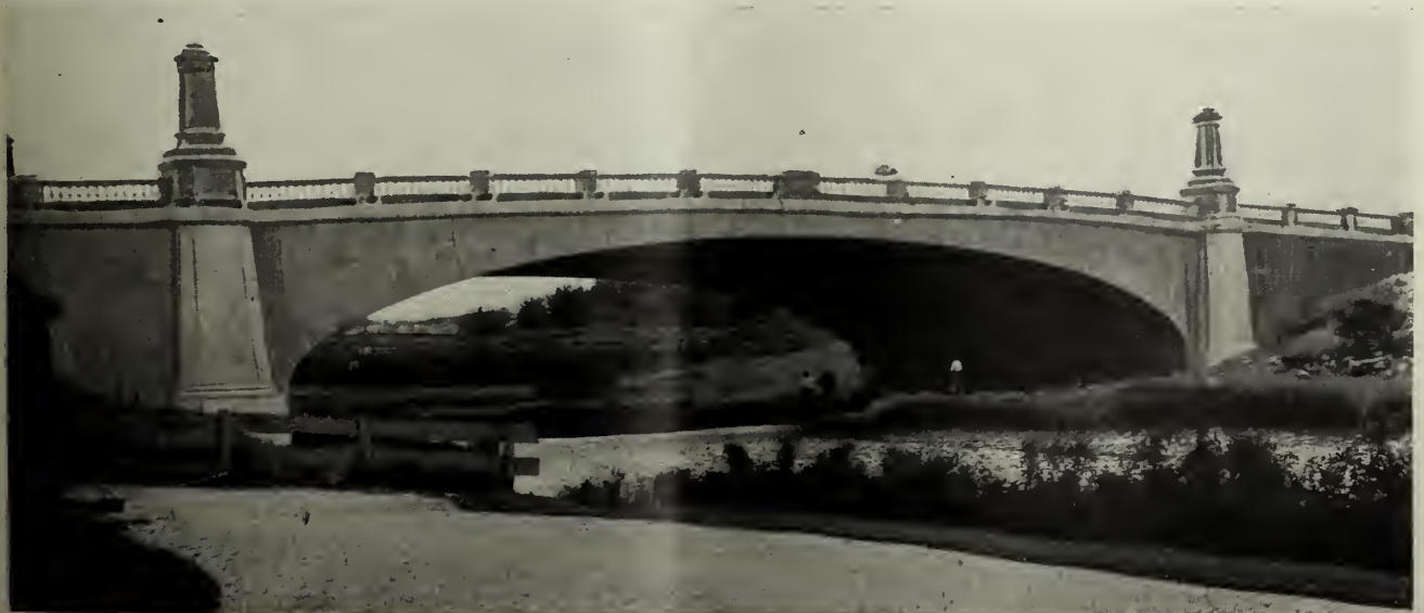
PARK AVENUE BRIDGE, ESSEX COUNTY, N. J., PARK SYSTEM.
