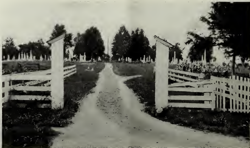
THE MAIN ENTRANCE—BEFORE.
