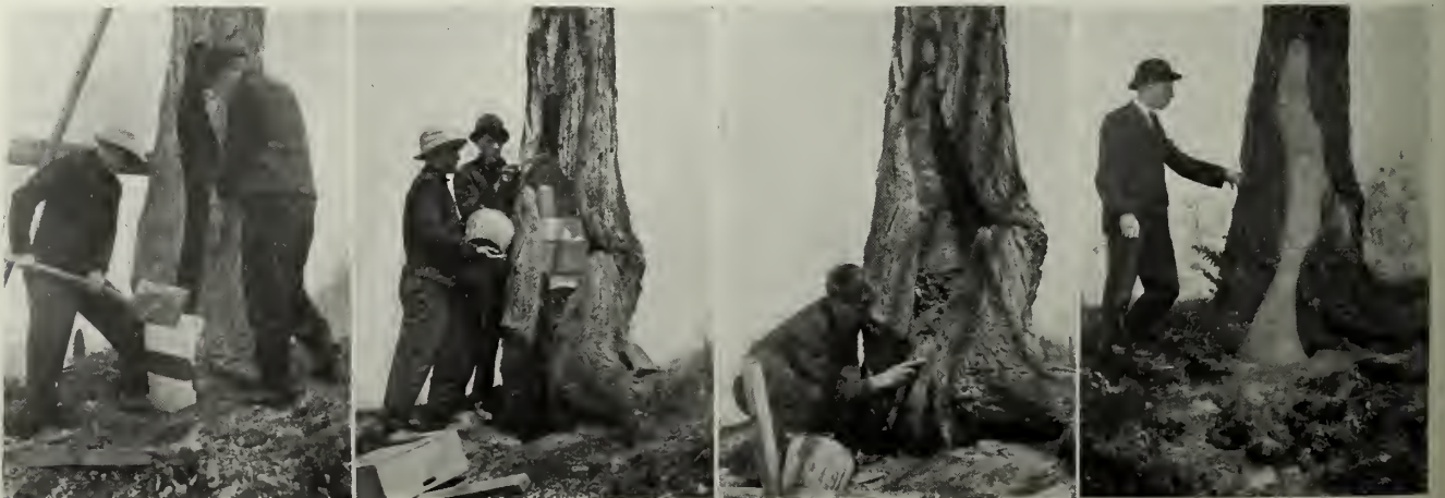
Tree Cleaned and Cement being tamped in.
