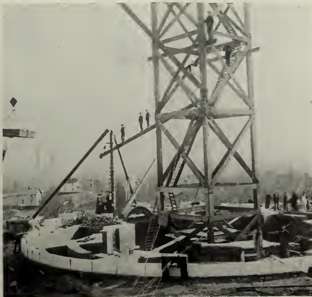
BEGINNING WORK ON THE MAIN STRUCTURE. Showing foundation and tower derrick.
