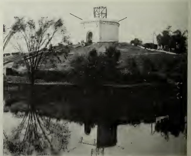
THE MAUSOLEUM AND APPROACHES. View from the east, showing main and east approaches; a part of the granite of east approach in position. Note reflection in water.
