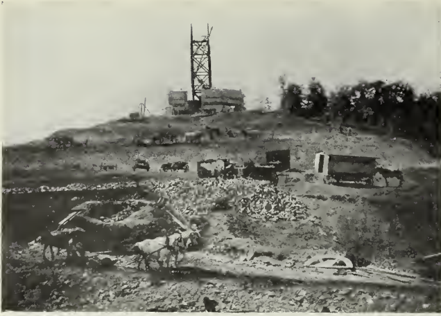
GRADING THE TERRACE.
