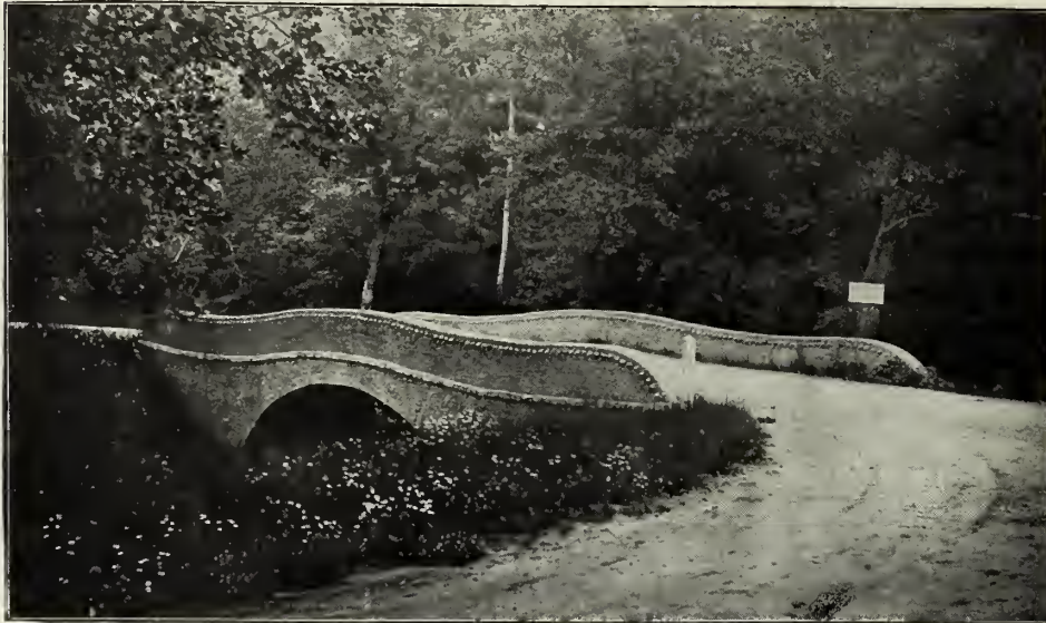
STYLISH LITTLE CEMENT AND PEBBLE BRIDGE. Crossing a tributary of Rock Creek in Rock Creek Park. Cost $4,200.
