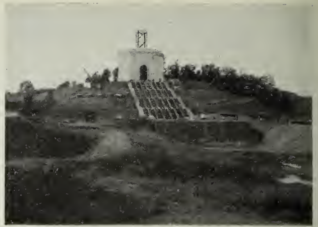
THE TERRACE, PARTLY GRADED.
