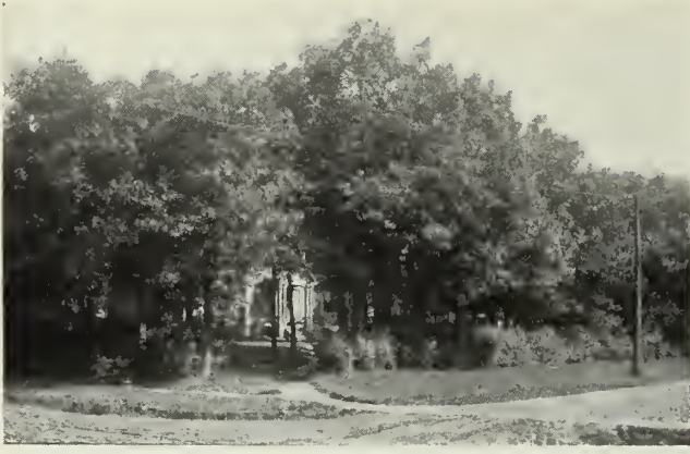
GROUNDS OF EAST SIDE SCHOOL. Menomonie, Wis.
