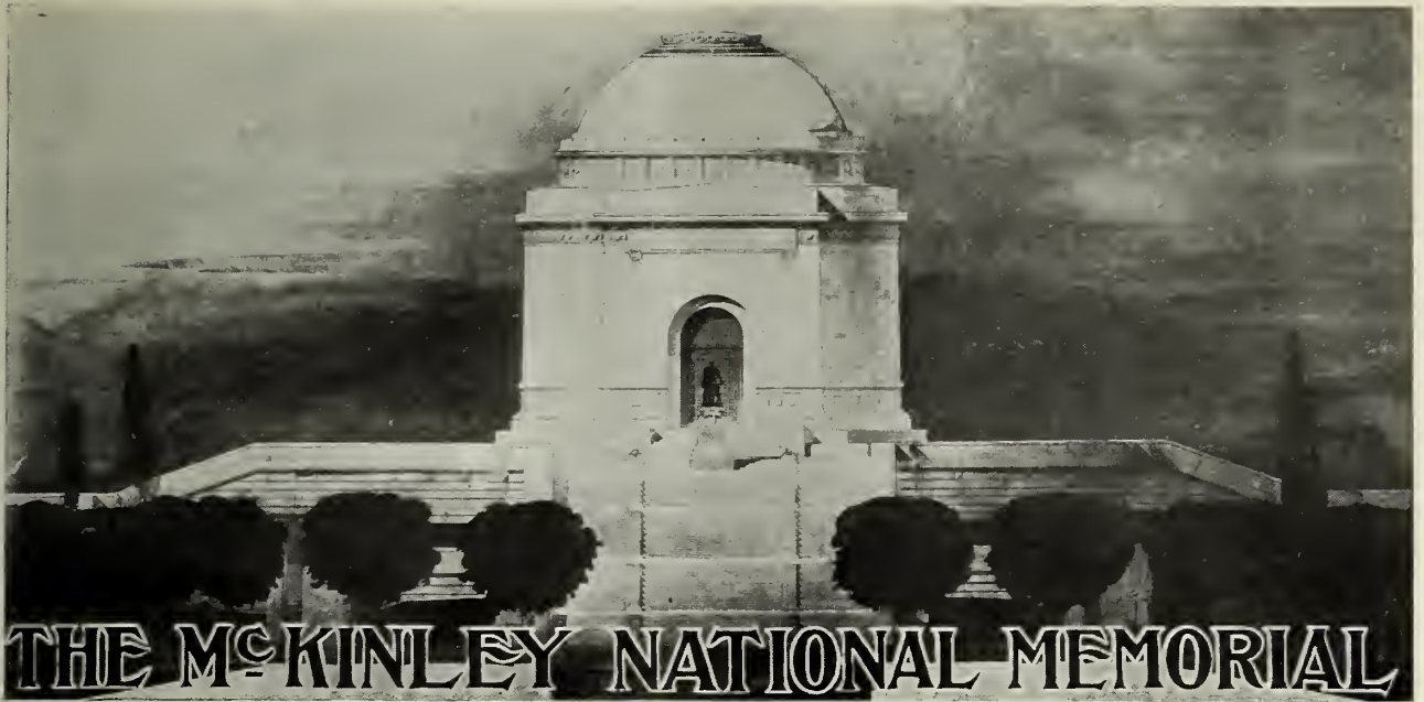
FRONT ELEVATION OF MCKINLEY NATIONAL MEMORIAL, CANTON, O.
