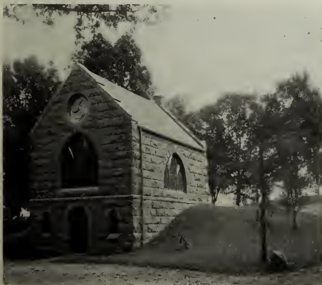
REAR VIEW OF CHAPEL AND VAULT. Jamestown, N. Y.
