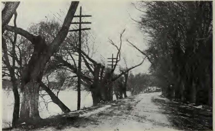
STREET TREES CUT BY LINEMEN.
