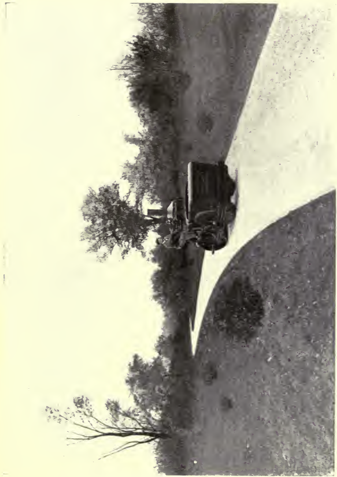
FIG. 16.—Park Walk. Drainage in Grass Cutters. Rolling being Done by Special Tandem Roller.
