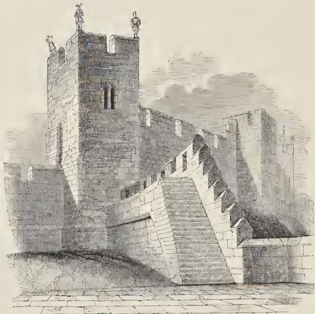
THE ARMOURER'S TOWER.
