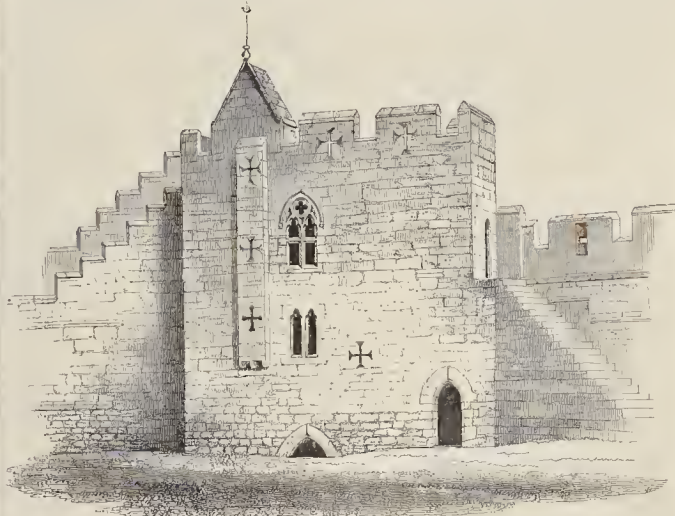
THE CONSTABLE'S TOWER.
