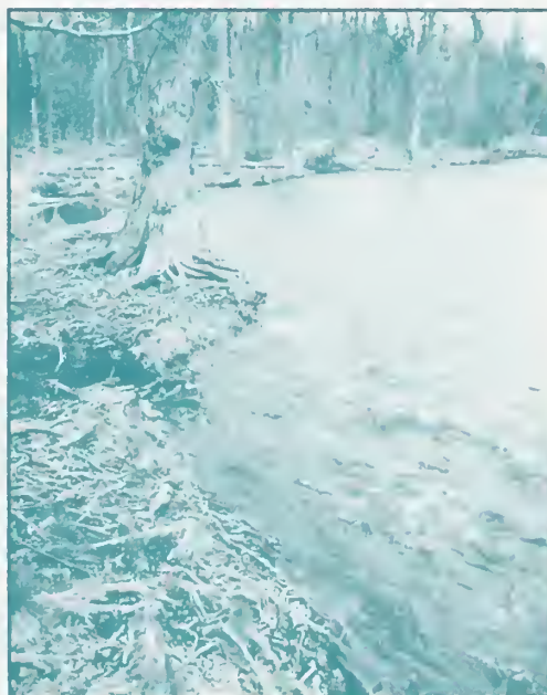
Eroded soils at the Russian River expose tree roots
