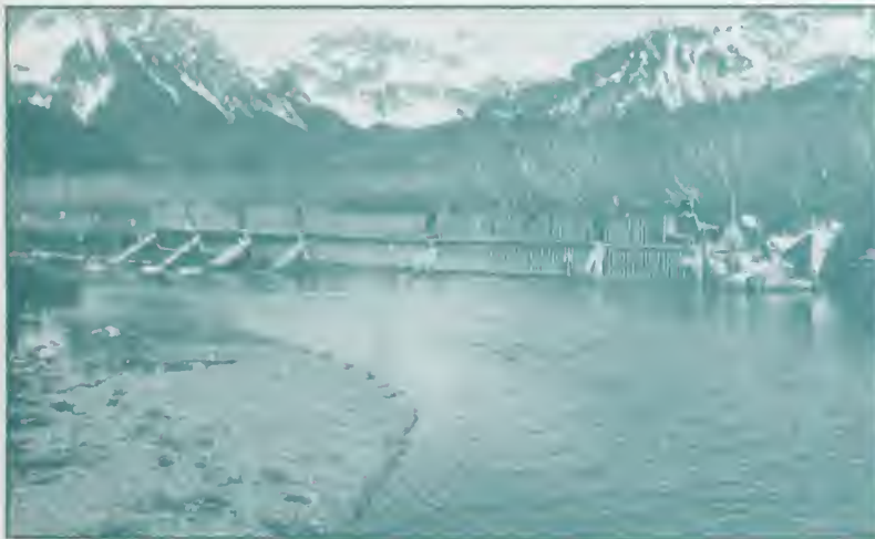
The Cordova Ranger District, with ADF&G, installed a full-capture weir on the Mile 18 system to assess coho production.
