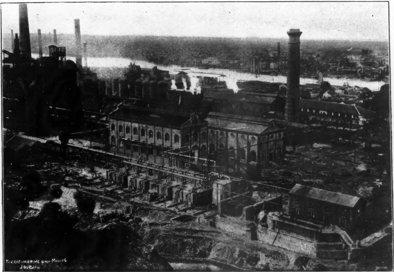
GENERAL VIEW OF THE IRON AND STEEL PLANT AT HANYANG, CHINA
