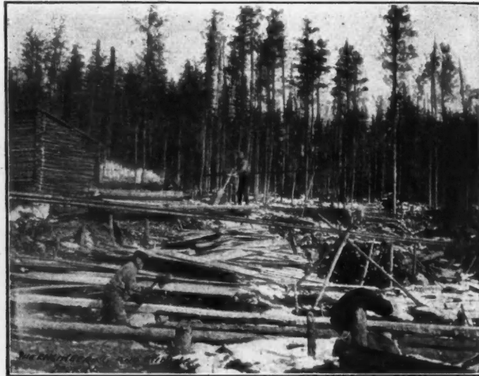
LUMBER FOR POWERHOUSE MADE WITH WHIPSAW AND BROAD-AXE
