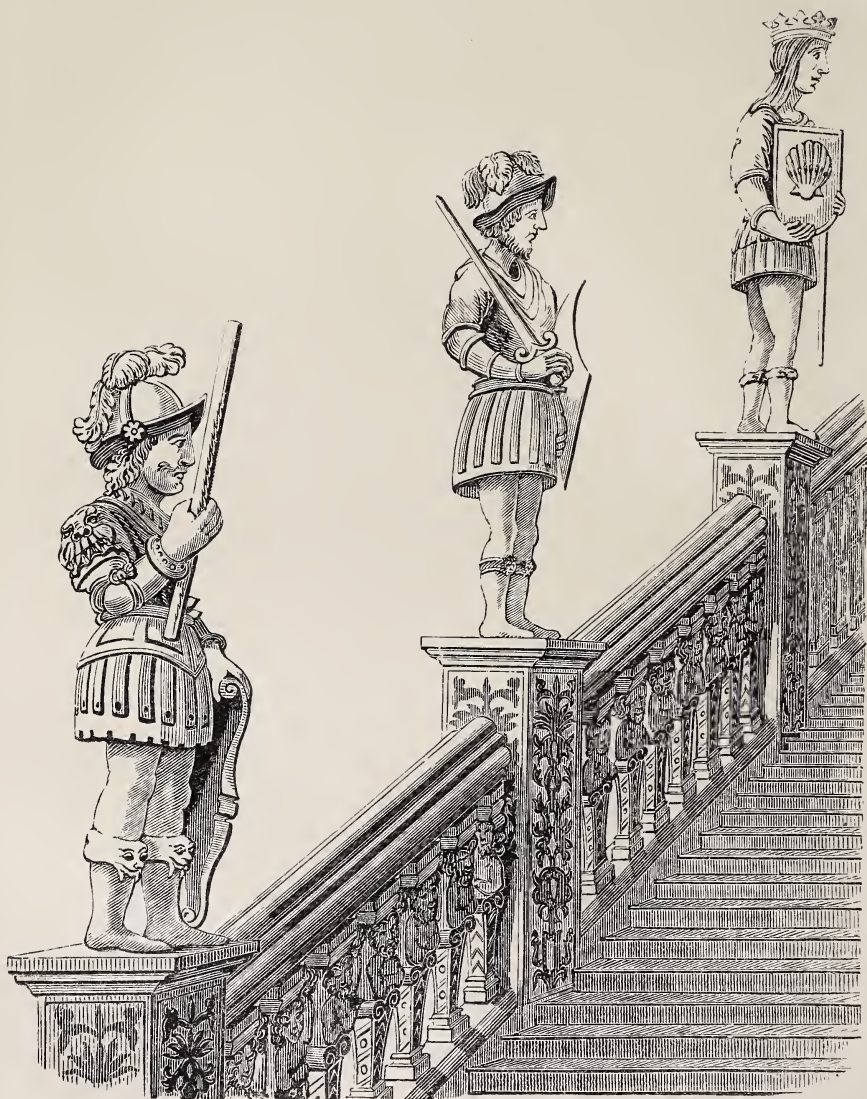
PART OF THE GREAT STAIRCASE AT HARTWELL HOUSE.
