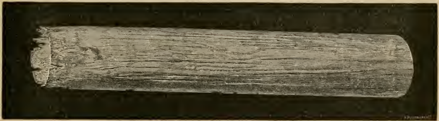
A CORRODED GAUGE GLASS.
