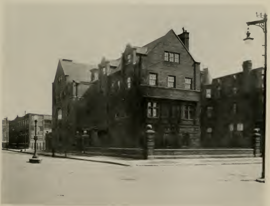
AN ABANDONED RESIDENCE IN THE PRAIRIE AVENUE BLOCK WITH A FACTORY IN THE REAR
