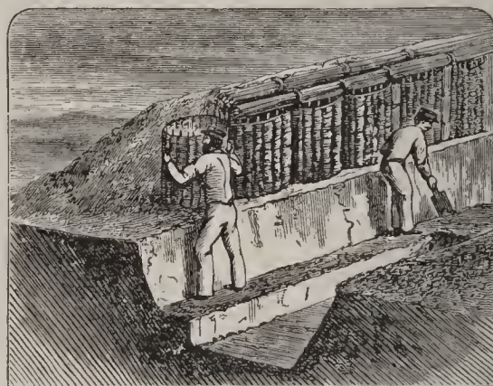
Part of Trench with Gabions and Fascines.
