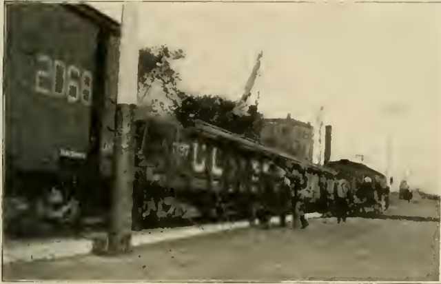
UNLOADING LONG RAILS.
