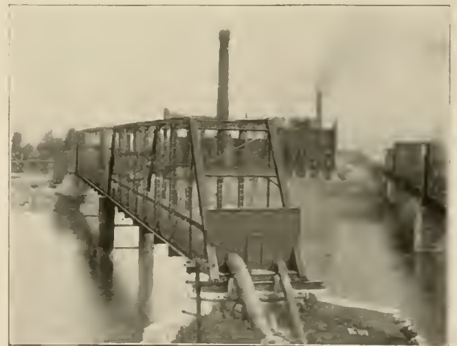
AQUADUCT BRIDGE OVER THE KANSAS RIVER.
