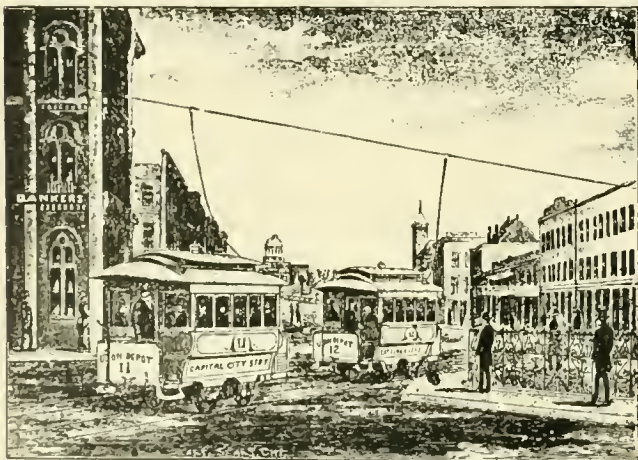
ONE OF THE EARLY INSTALLATIONS.
