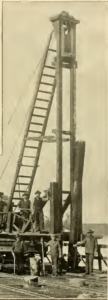
ELECTRIC PILE DRIVER, SEATTLE.
