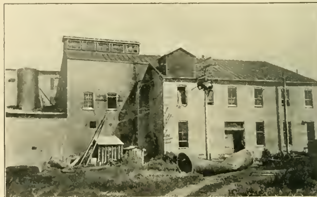
POWER HOUSE AFTER THE STORM.
