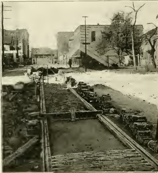
LAYING BUCKLAND PAVING BLOCKS.
