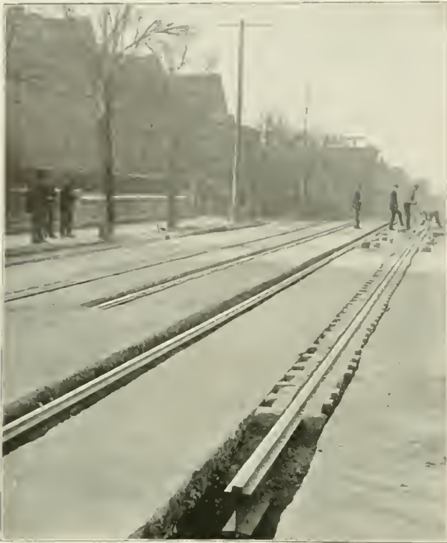
TRENCH CONSTRUCTION NORTH AMERICAN RAILWAY CONSTRUCTION CO.
