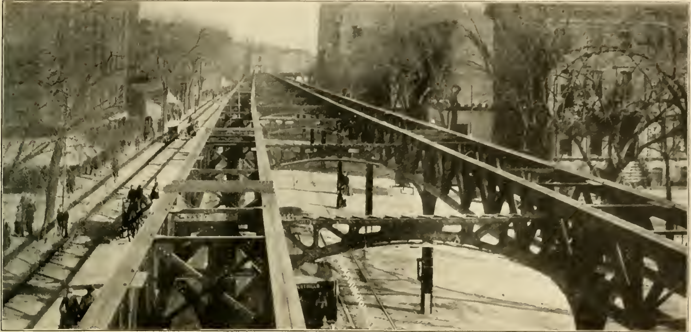
FIG. 7—STRUCTURE AS ERECTED IN WIDE STREETS.
