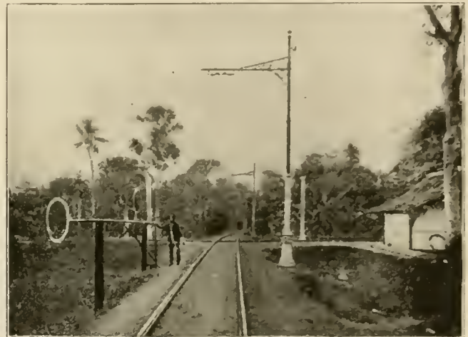
FIG. 3—TRACK SHOWING LINE CONSTRUCTION.
