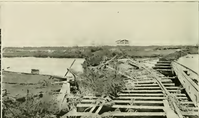
BRIDGE AT 43d ST. AND AVE. R.
