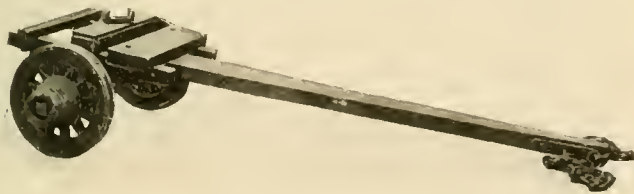
FIG. 49—TRUCK USED IN REMOVING WAGONS.
