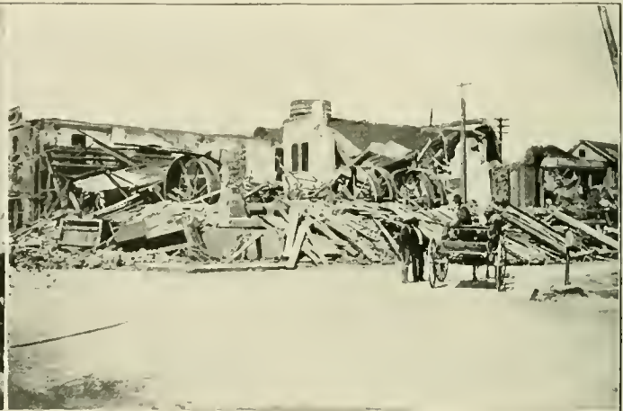
WRECK OF POWER HOUSE.
