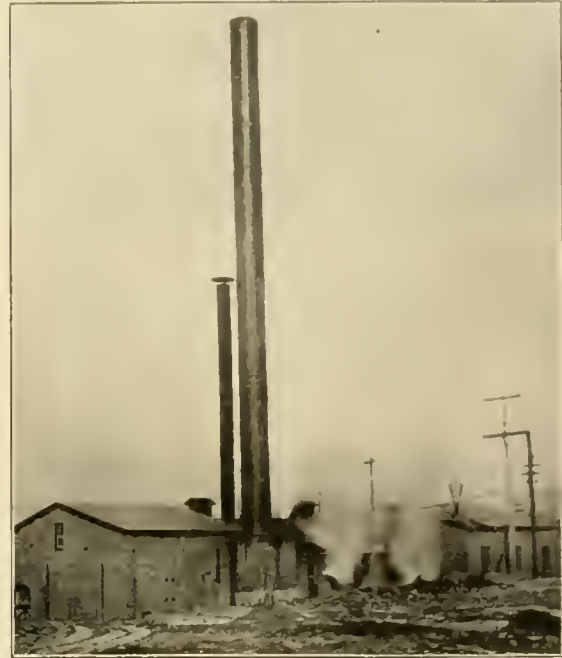
FIG. 2—EXTERIOR OF POWER HOUSE.
