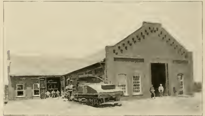
GENERAL OFFICES AND CAR HOUSE.
