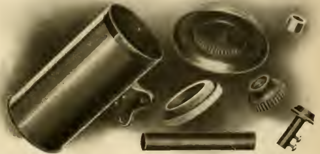
WOOD'S LIGHTNING ARRESTER.
