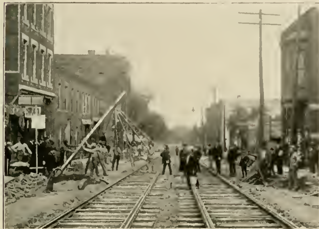
WORK OF ELECTRIC INSTALLATION CO. ON 14TH ST.
