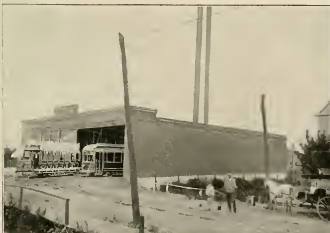
POWER STATION AND CAR HOUSE.
