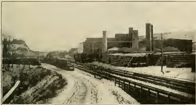
PLANT OF POTOMAC TERRA COTTA CO.
