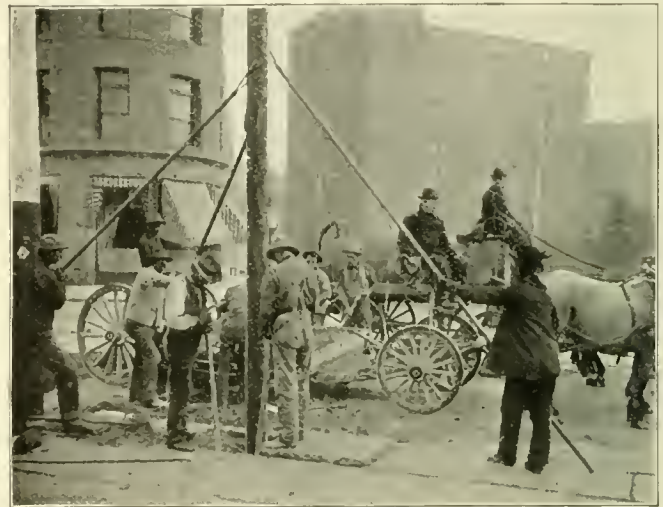
CONCRETE WAGON AND CREW.
