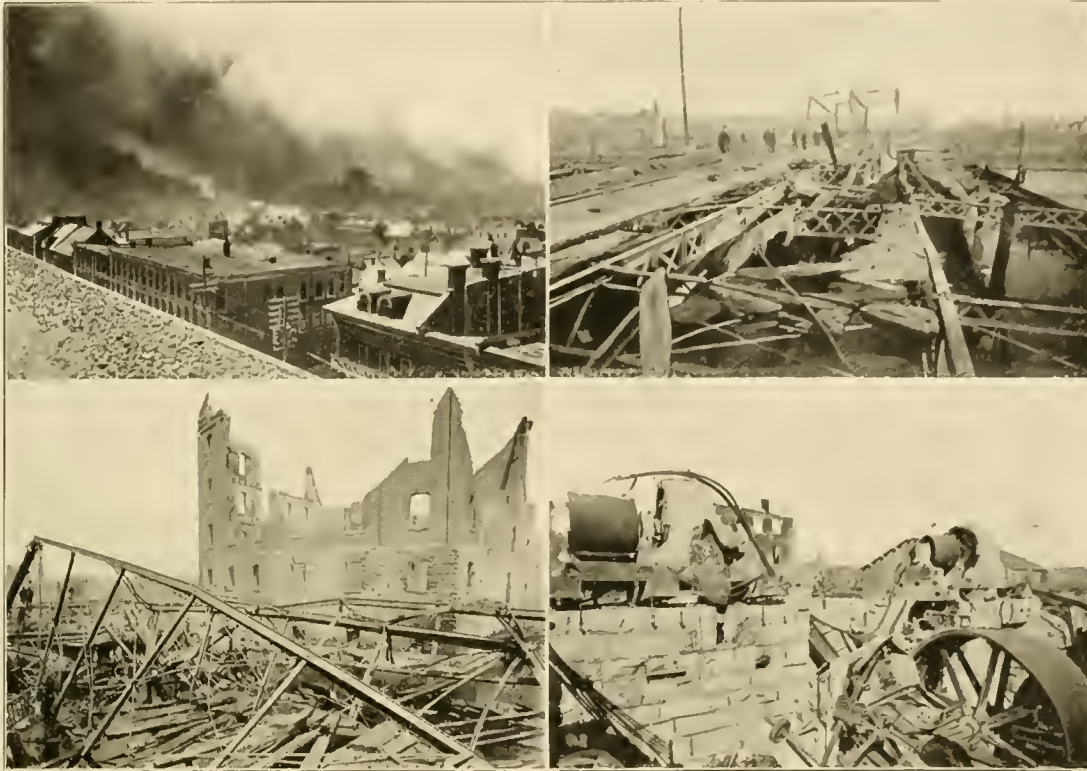
GENERAL VIEW FROM HOTEL CECIL. RUINS OF IRON BRIDGE No. 2.
