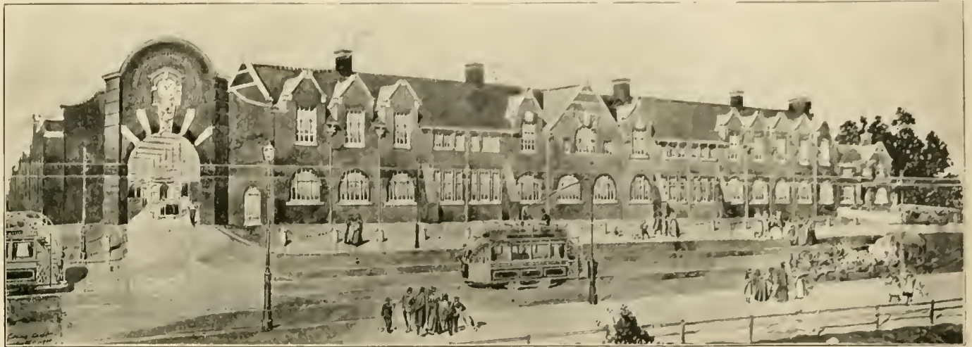
EXTERIOR OF QUEEN'S ROAD CAR SHED, MANCHESTER (ENG.) TRAMWAYS.
