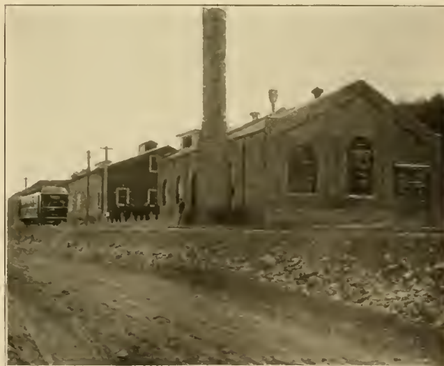
FIG. 2 EXTERIOR OF POWER HOUSE.
