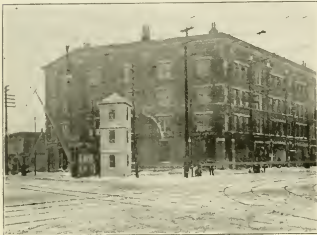
SWITCH TOWER AT WILLSON AND EUCLID AVES., CLEVELAND.
