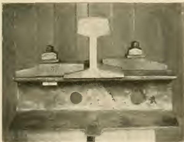
FIG. 2—FASTENINGS FOR REROLLED STEEL TIES.
