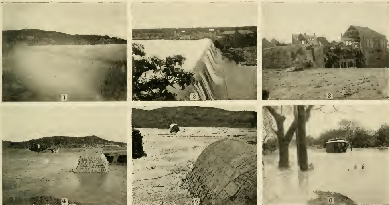
THE AUSTIN DAM AND VIEWS AFTER THE FAILURE.
