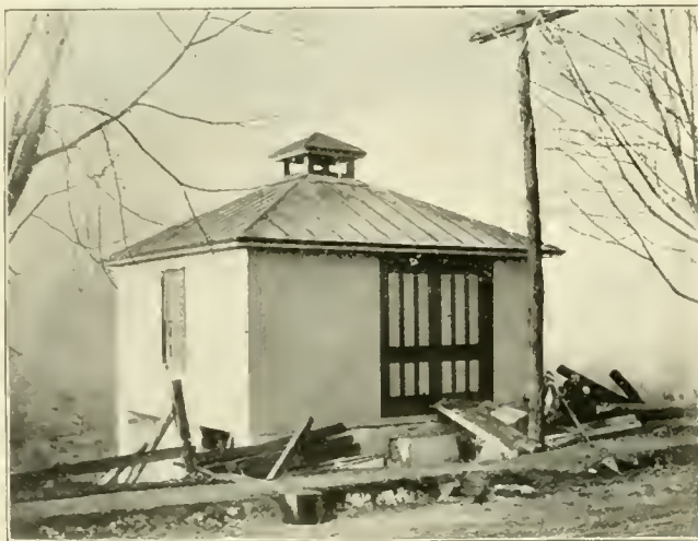
FIG. 6—EXTERIOR OF SUB-STATION.
