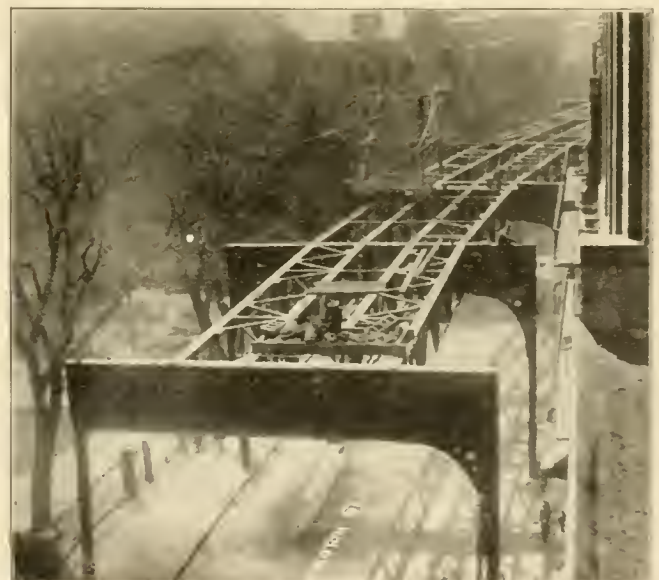
FIG. 10—PLATE CROSS GIRDER CONSTRUCTION.
