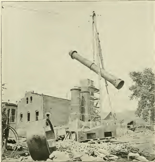
FIG. 4—ERECTING BOILERS AND STACK OF NEW PLANT.
