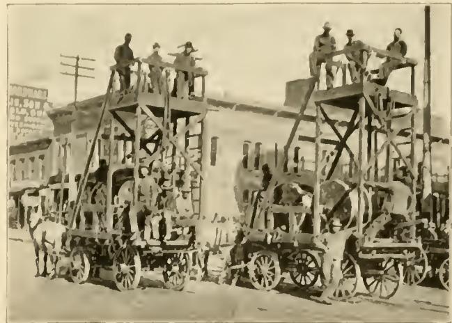
TOWER WAGONS AND CREWS.
