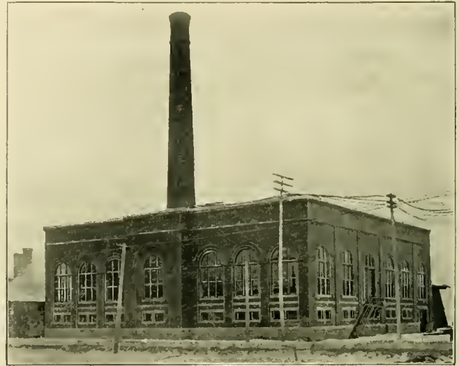
FIG. 6—POWER HOUSE, PORTLAND R. R.
