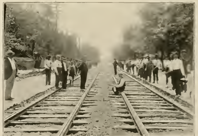
TRACK ON BROADWAY, ELECTRIC INSTALLATION CO.
