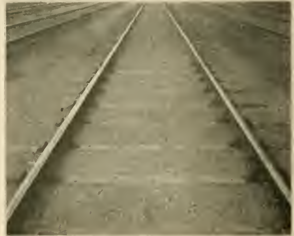
FIG. 3—TRACK LAID WITH STEEL TIES.
