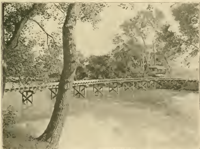
BRIDGE OVER ARKANSAS RIVER.
