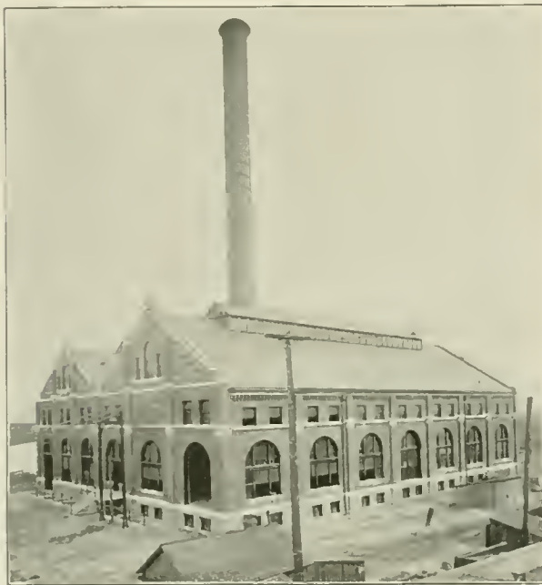
EXTERIOR OF KAW RIVER STATION
