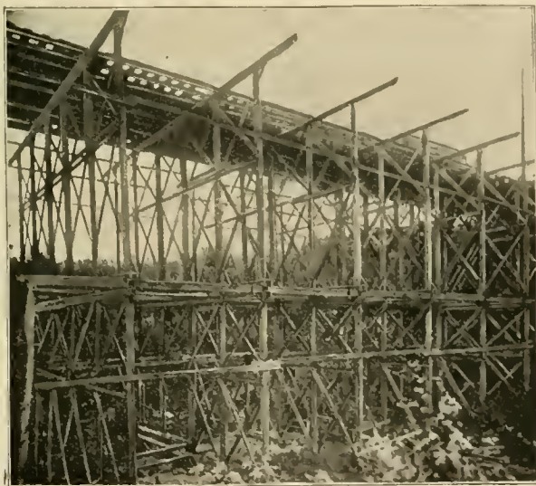
FIG. 4—BRIDGE FROM BELOW.
