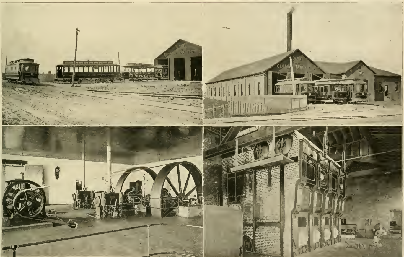
POWER HOUSE AND CAR BARN OF THE OHIO CENTRAL TRACTION CO., GALION, O.
