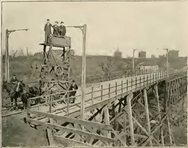
AGNES AVE. TRESTLE 1888.
