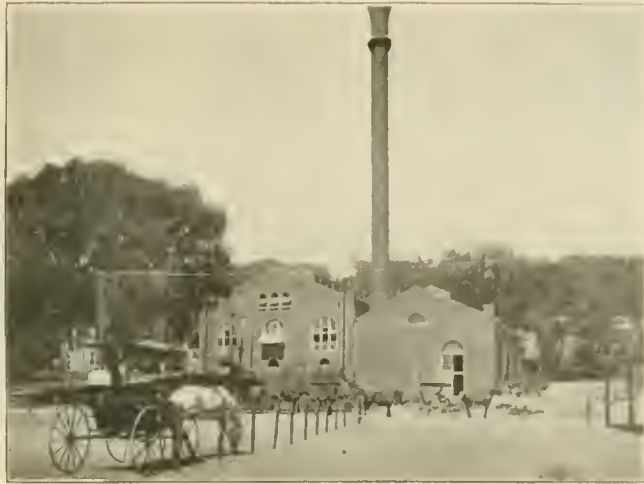
POWER HOUSE, EDGEWATER.
