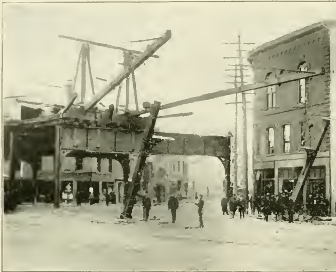
FIG. 12-ERECTING COLUMNS.
