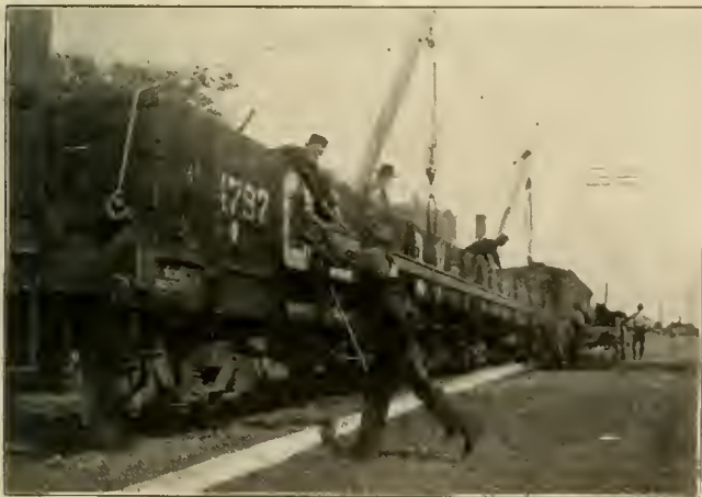
UNLOADING LONG RAILS.
