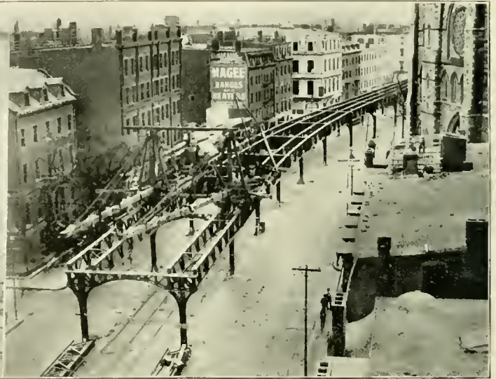
FIG. 13-ERECTING STRUCTURE.
