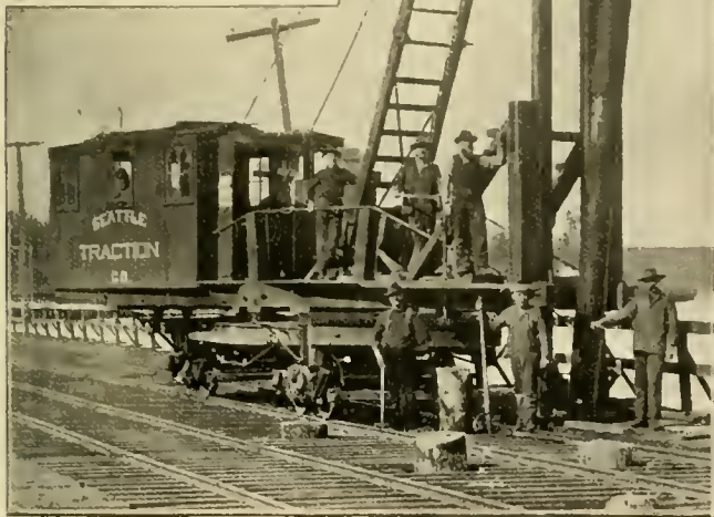
ELECTRIC PILE DRIVER, SEATTLE.
