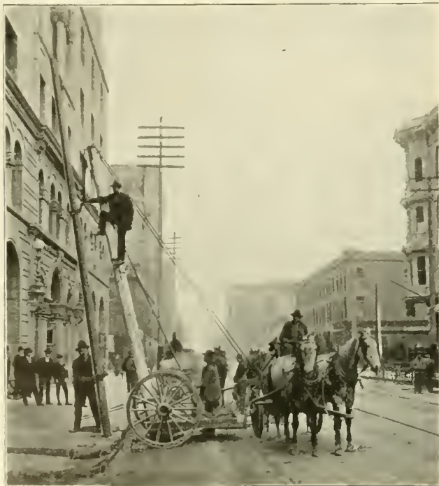
DERRICK WAGON FOR SETTING POLES.
