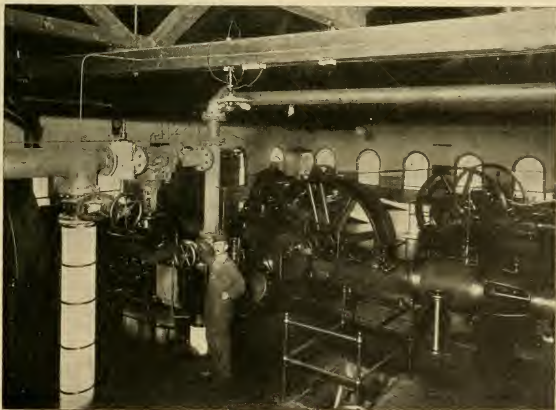
GENERAL VIEW OF POWER HOUSE, HAMPTON.
