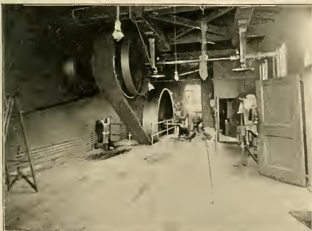
FIG. 2—ENGINE IN FIRST POWER HOUSE.
