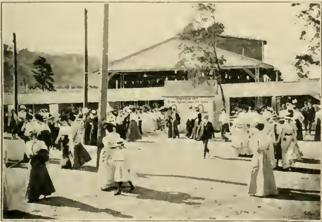
EXTERIOR, SHOWING ARRANGEMENT OF EXITS.
