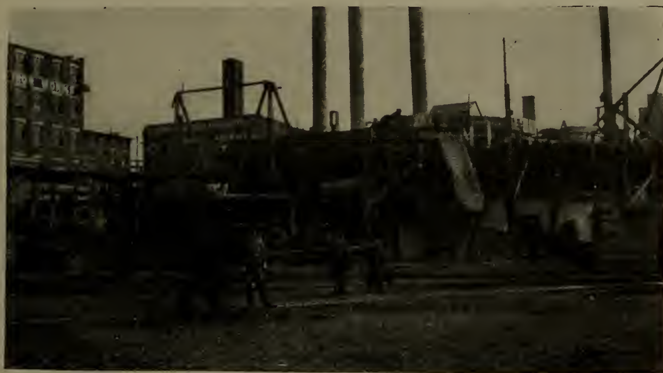
FIG. 7.—Manhattan Power House for P.R.R. North River Tunnels.
