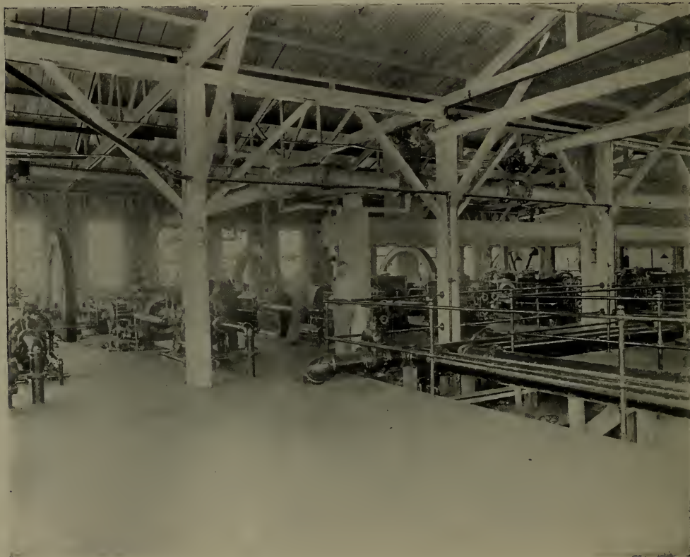
FIG. 8.—Interior of Weehawken Power House for P.R.R. North River Tunnels.
