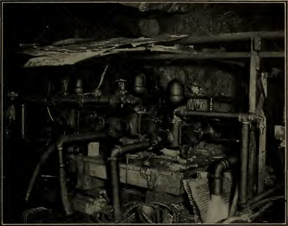
Battery of Cameron Pumps installed in "Belmont" Tunnel, under East River, under Man-O'-War's Reef.
