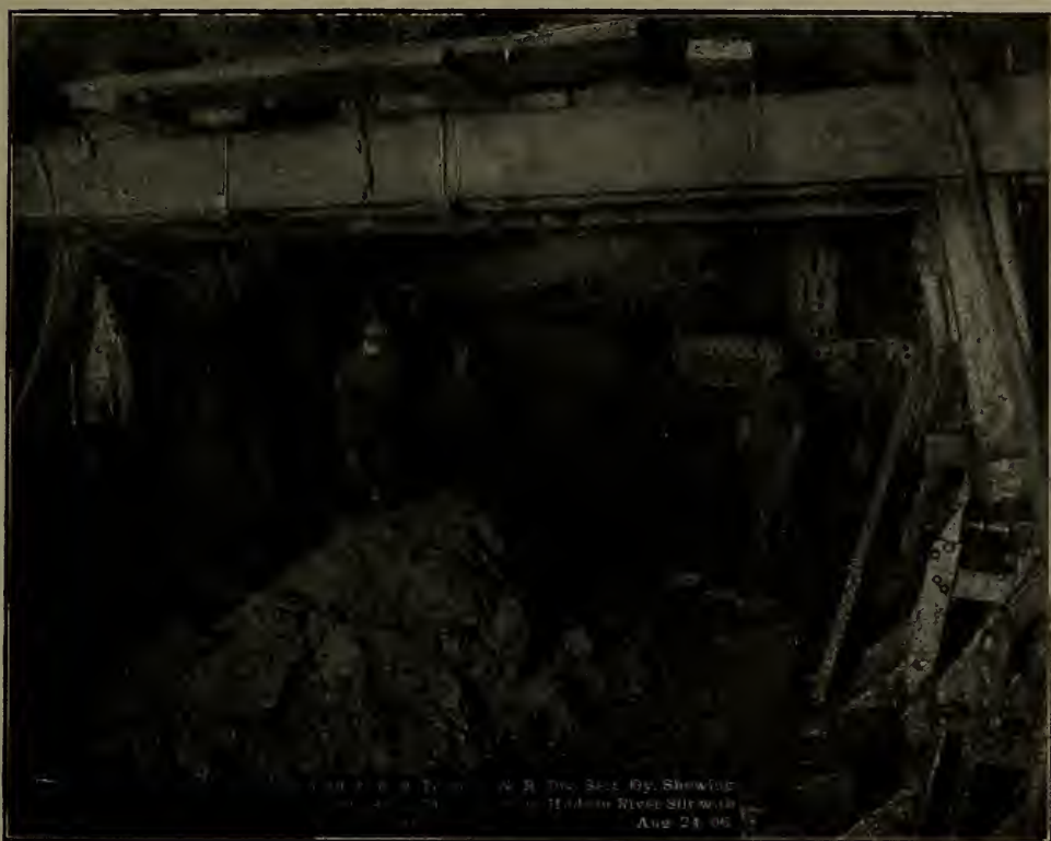
Interior of Shield in P.R.R. North River Tunnel, Showing Silt Entering Through One Open Door.
