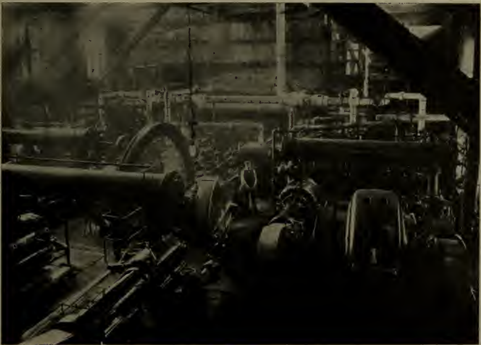
FIG. 3.—Interior of Power House for P.R.R. Terminal Excavation.
