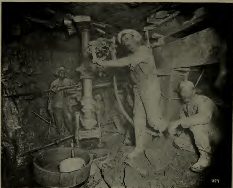
Ingersoll-Rand Rock Drills in Heading of One of the East River Subway Tunnels.
