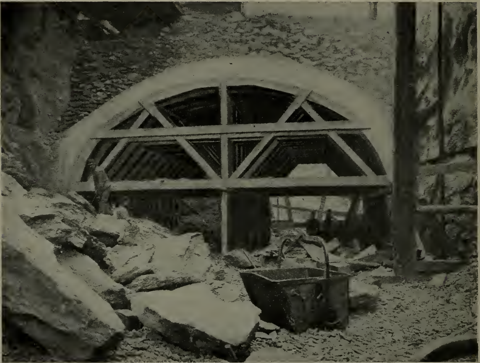
Concrete Arch Subway Construction in Open Cut.
