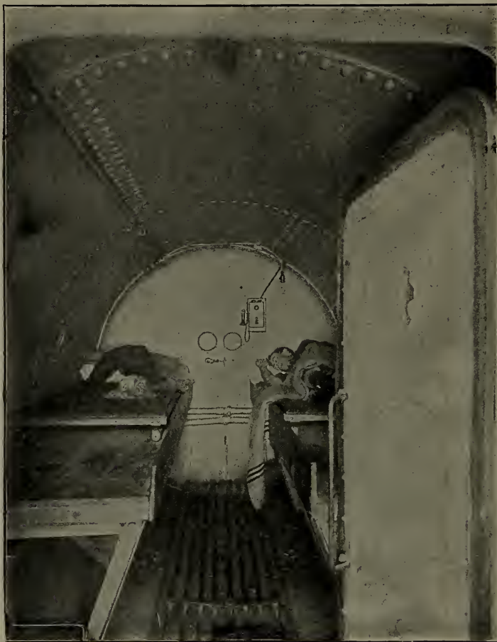
FIG. 1.—Interior of Medical Air Lock.
