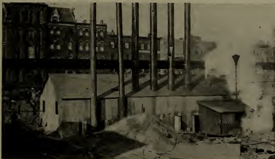
FIG. 1.—Temporary Power House, Pennsylvania Terminal.
