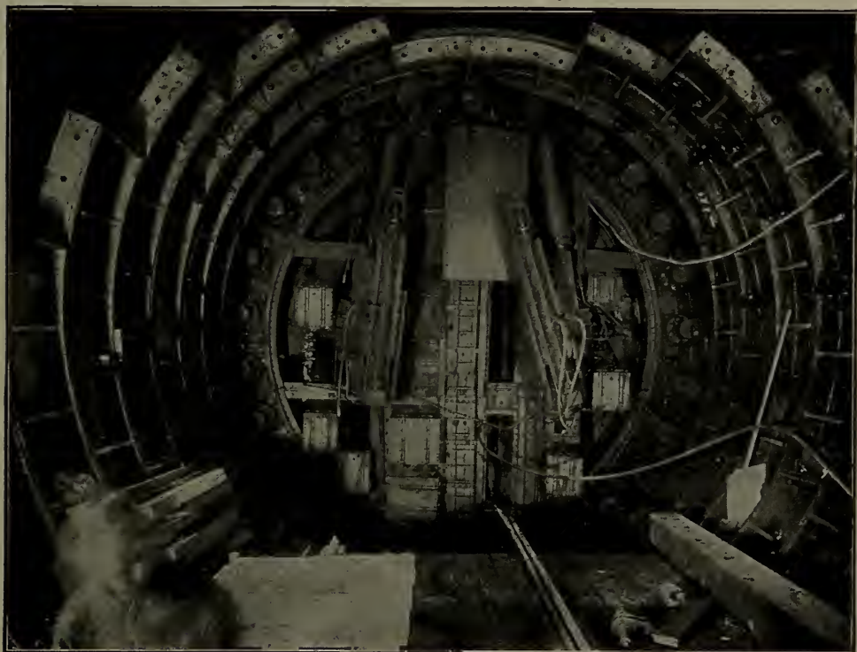
Rear of Shield showing Complete Fittings.
