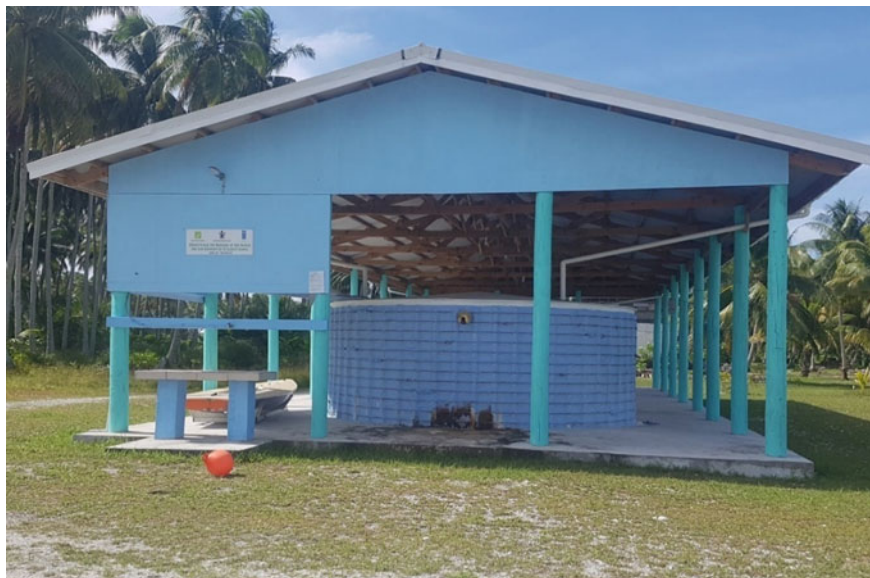
Fig. 10.3 Community water tank and catchment roof on the atoll of Manihiki (©Melina Tuiravakai)
