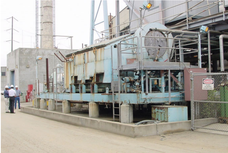
Fig. 8.2 An 817 m 3 /d flash evaporator c.1970 (© Tom Pankratz)
