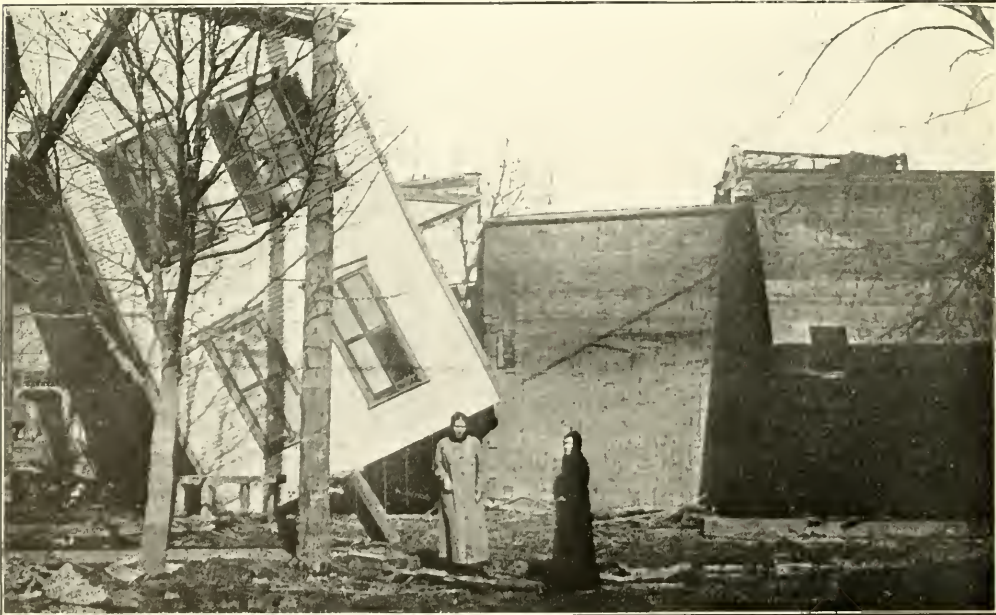
This is not an unusual sight, as almost every block in the city has houses in such disorder.
