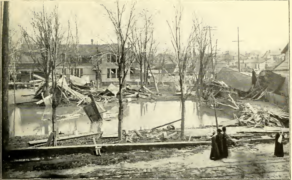
Flood Ruins on Third Street, near Mound, looking South.
