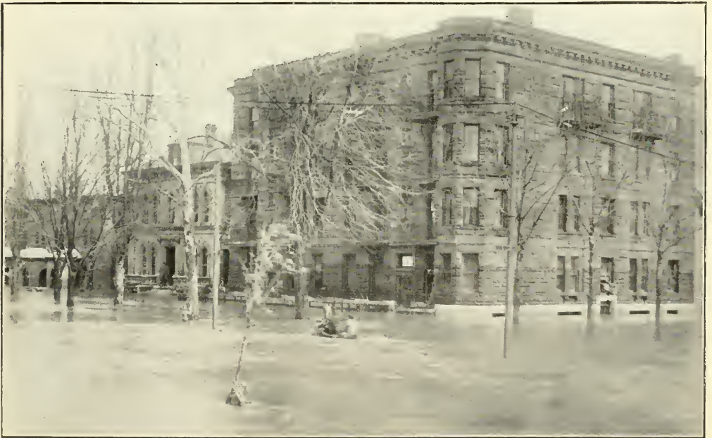
Receding water at the corner of Third Street and Robert Boulevard. Note the high water mark on the building.
