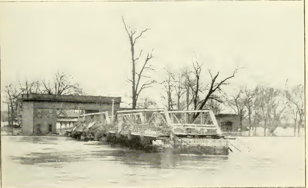
The White City Bridge.
