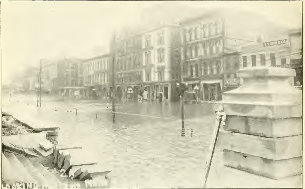
Receding Water in North Main Street.
