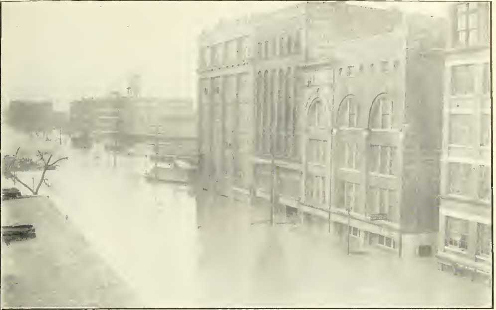
East Third Street from Wayne Avenue.
