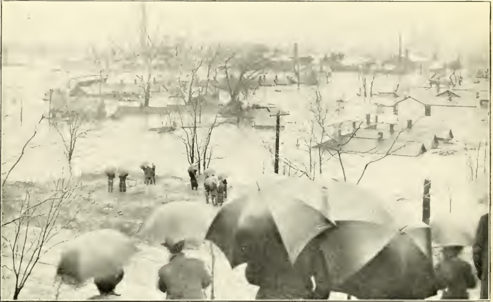
Looking North from the Fairgrounds, and West of Main Street at Apple. One-story cottages in distress.
