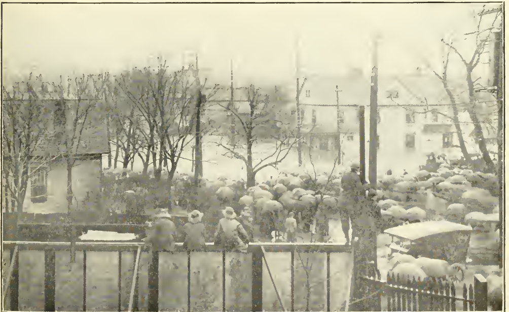
Corner of Main and Apple Streets. From which point, Mr. Patterson directed heroic rescue work.
