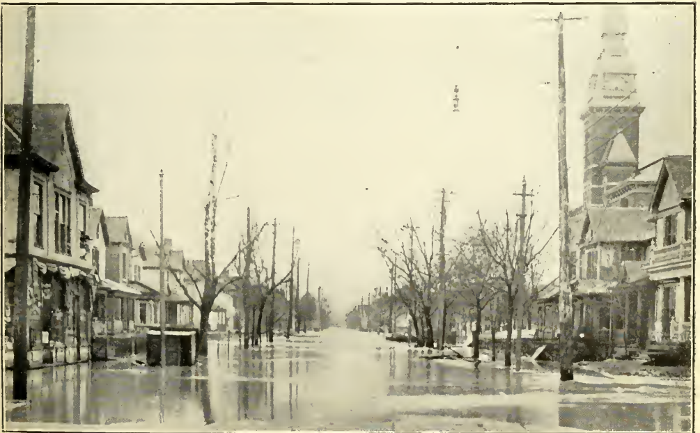
The Western Edge of the Flood on West Fifth Street Extended to Conover Street.
