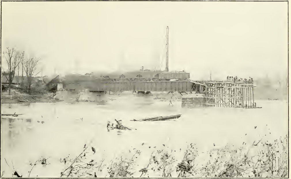
Repairing the Railroad Bridge.
