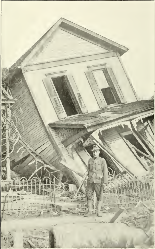
Wrecked House in North Dayton.
