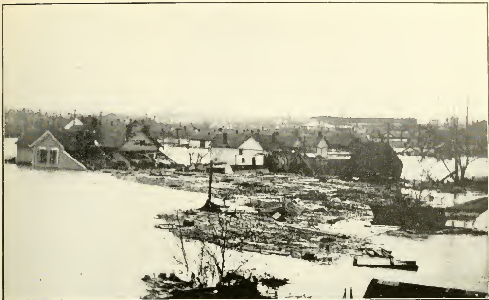
Another Scene of Destruction in North Dayton.
