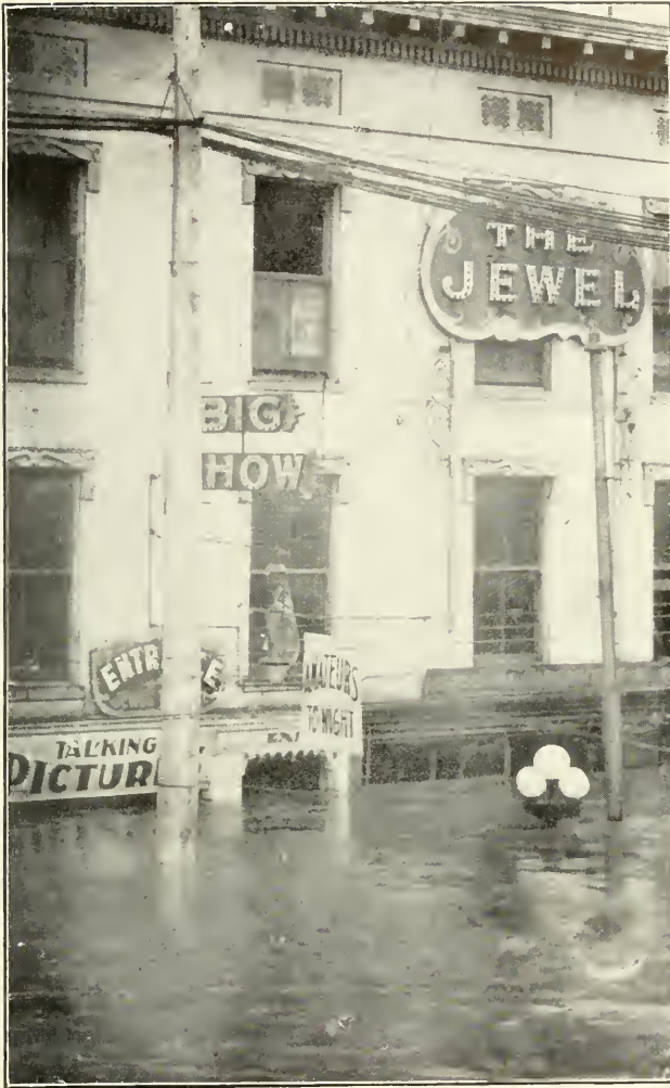
High water in South Jefferson Street.
