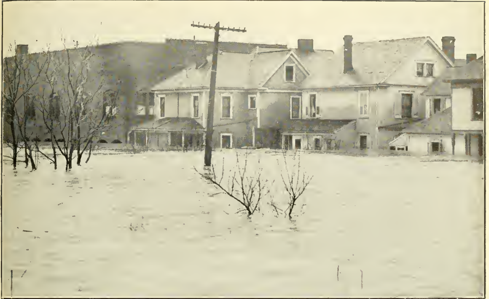
Rear of Grimes Street at Edgewater.
