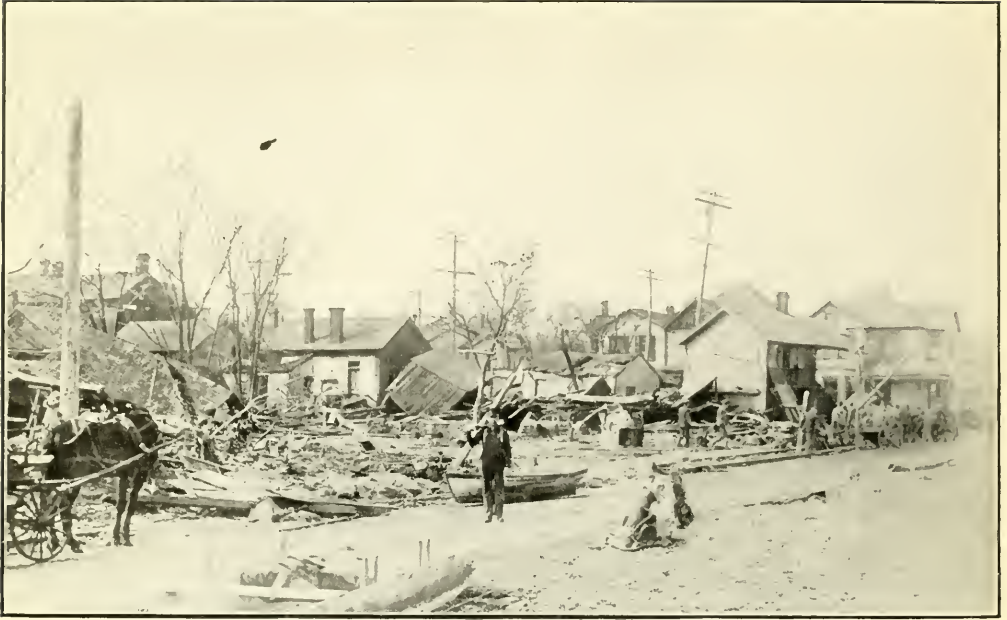
Some of the Destruction on Burns Avenue.
