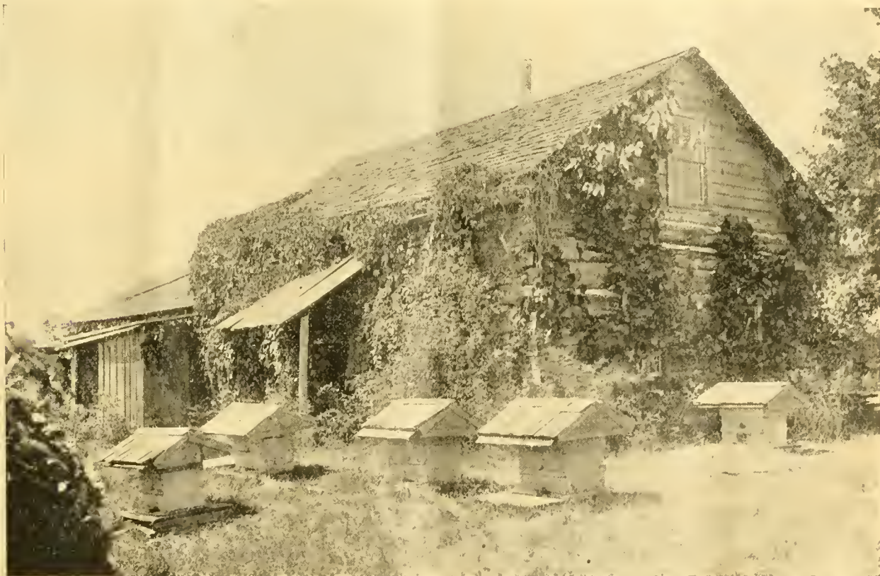
The Old Home of Two Lady Pioneer Bee-Keepers in Michigan—From the Bee-Keepers' Review.
