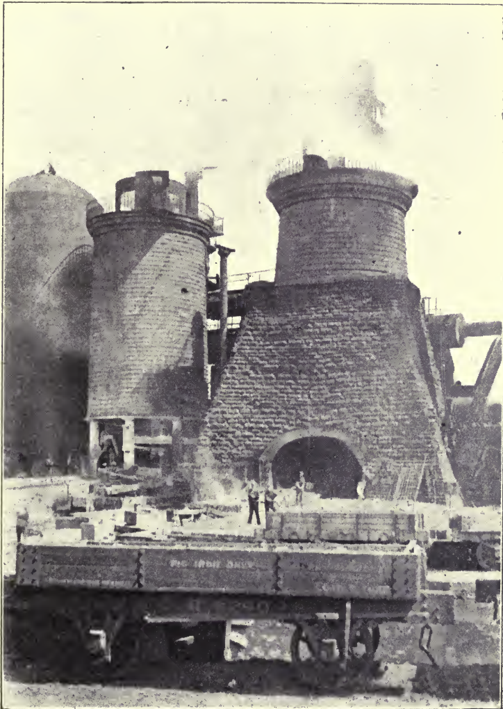
FIG. 77.—No. 1 Furnace, Gartsherrie. Erected 1836; demolished 1896.
