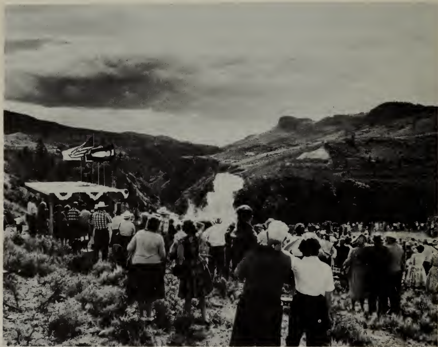
The first rock is blasted from the canyon walls of Gunnison River, Colo., at ground-breaking ceremonies for Blue Mesa Dam.
