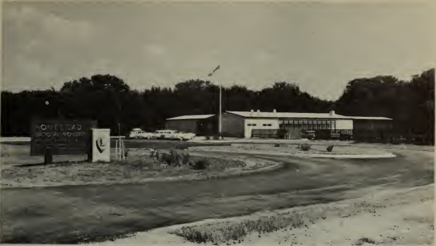
New visitor centers were constructed in nine National Park Service areas. One of these was dedicated at Homestead National Monument, Nebr., on June 10, 1962.
