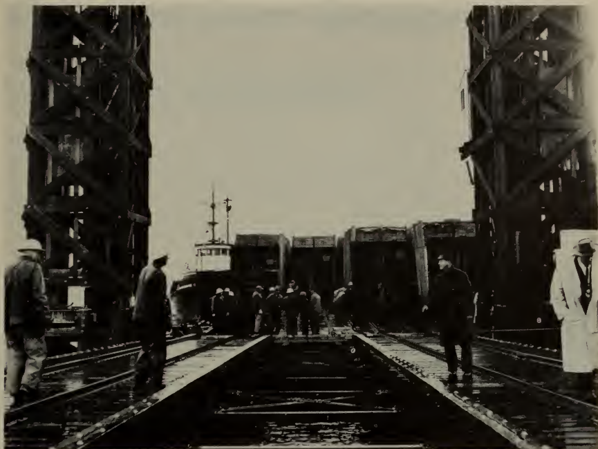
The arrival of Canadian National Railways barges started in May 1962, bringing new service and substantial economies
