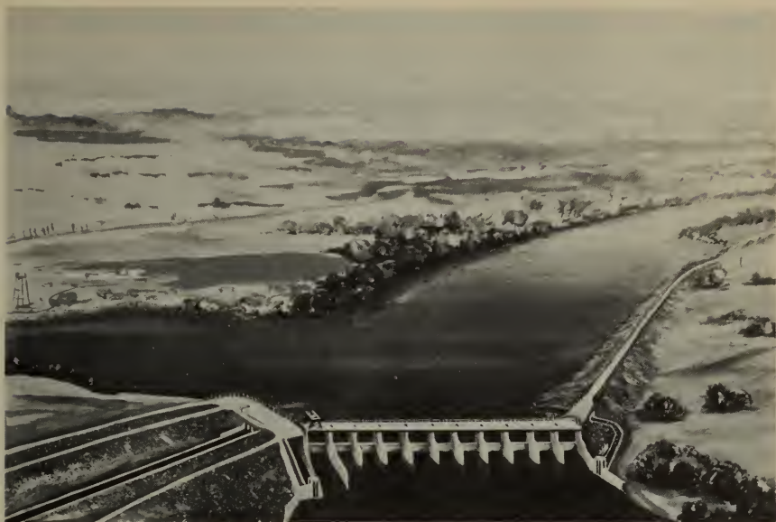
Red Bluff Diversion Dam, now under construction on the Sacramento River as part of the Central Valley project, California—artist's conception.
