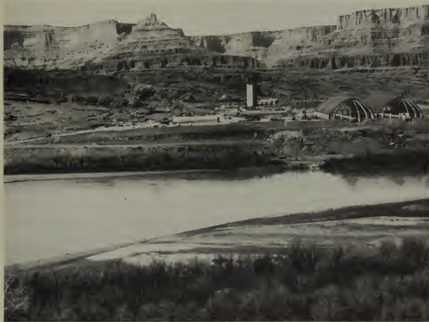
Texas Sulphur Co.—potash mine development on Colorado River at Kane Springs Wash, Utah.
