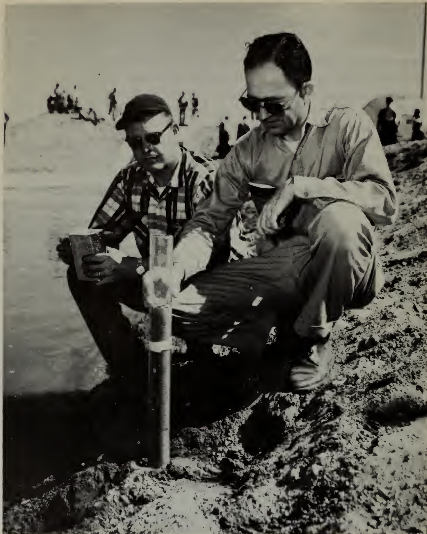
Engineers test wax emulsion sealant to reduce seepage loss from irrigation canal, Eden project, Wyoming.
