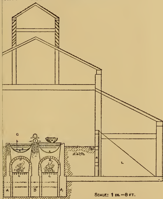
SECTION OF KETTLE BLOCK.
