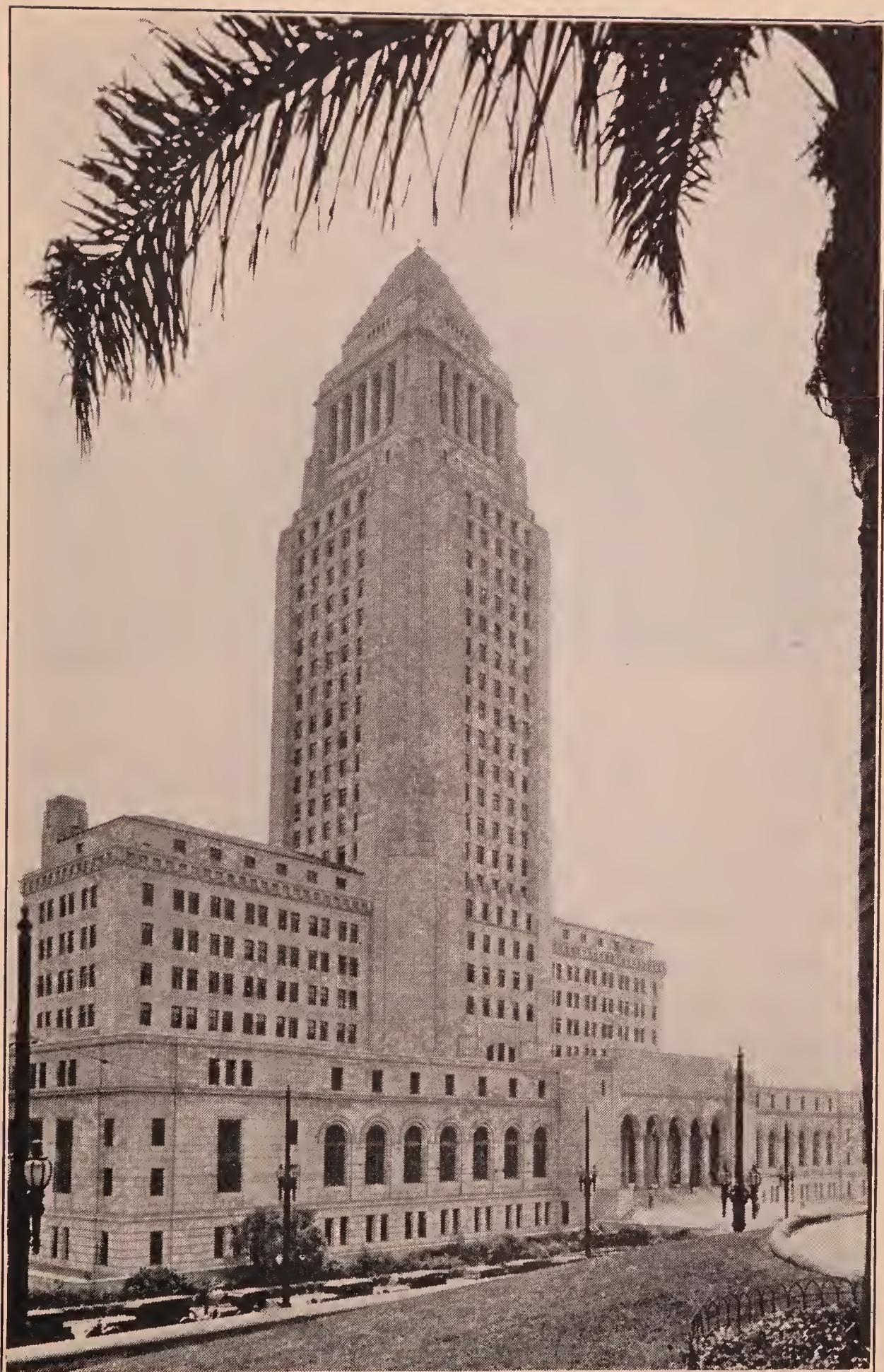
CITY HALL, LOS ANGELES
