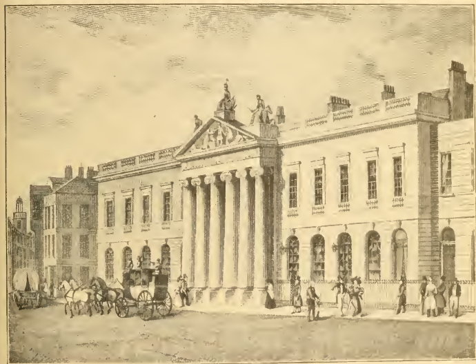
MANSION OF THE EAST INDIA COMPANY, LONDON.
