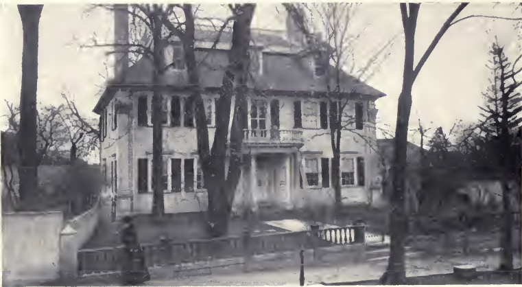
GOV. JOHN LANGDON HOUSE, 1784; PORTSMOUTH
