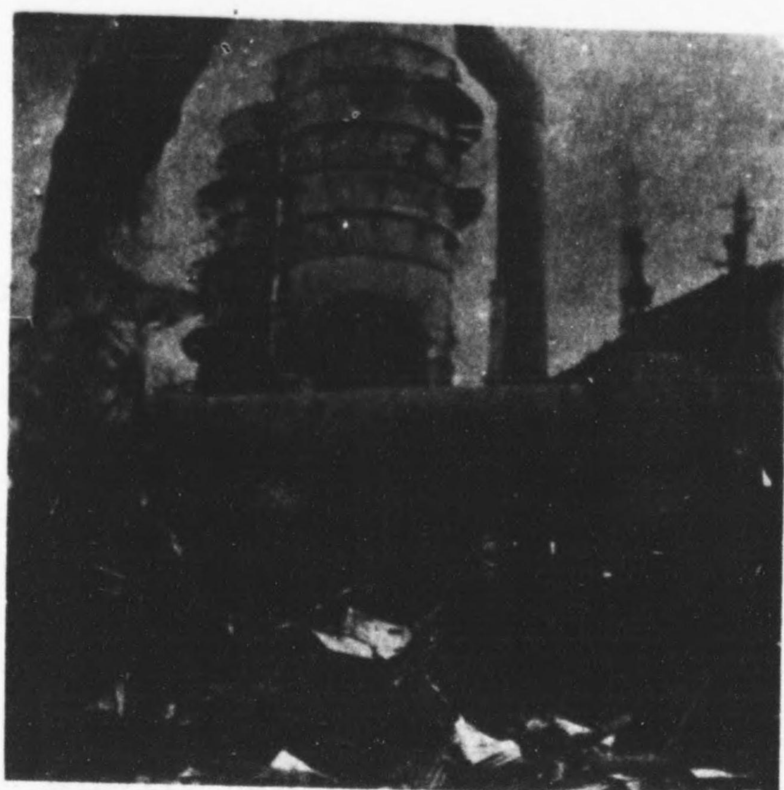
Figure 5. - Blast Furnace at Kamaishi Hit by U S Navy Shell
