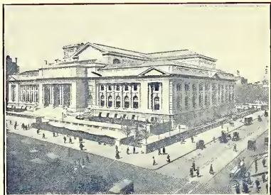
Public Library, Forty-second Street and Fifth Avenue, New York
