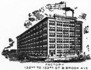
FACTORY 132 ND TO 133 RD ST & BROOK AVE
