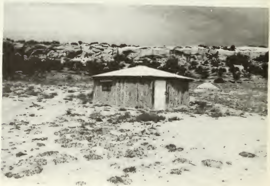
CM-186. Recent winter hogan still in use. The hogan has jacal style walls, conical tar paper roof, glass window, and door made from lumbered wood. (looking west)
