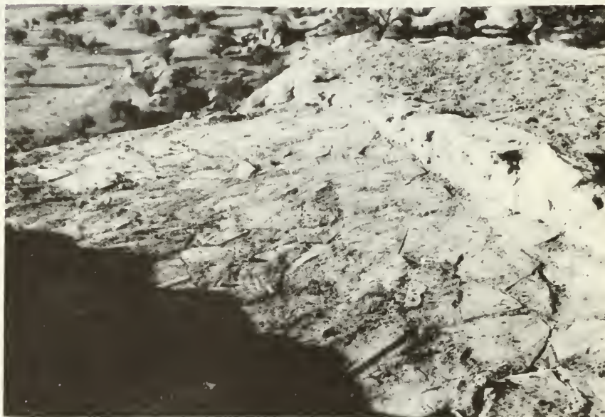
"After" stabilization; the reconstructed section of the roof on room 1. Note the sandstone slabs on the roof surface. (looking southwest)
