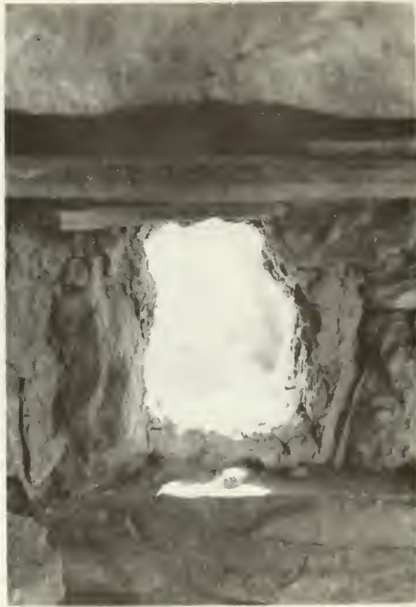
Loop-hole style window in the south-east corner of room 1. Note the adobe and sandstone slabs lining the window.
