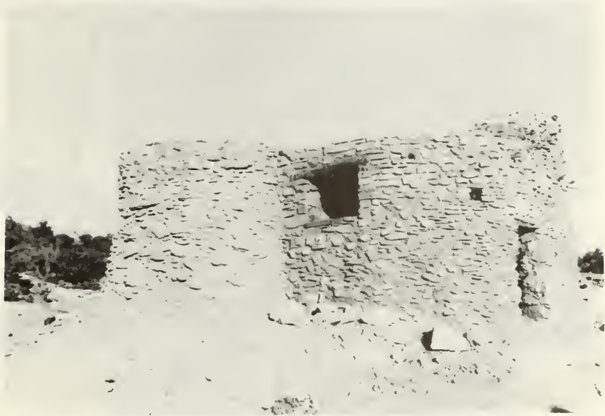
"After" stabilization; the south facing walls of CM-38. (looking northwest)
