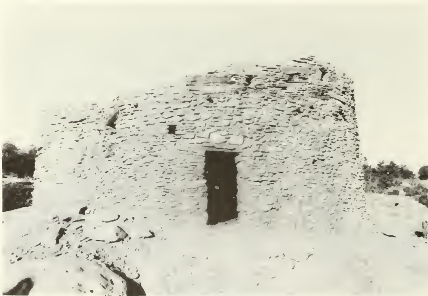
"After" stabilization; the east facing walls of CM-38. (looking west)
