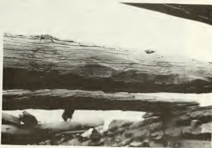
Close-up of an original viga showing trimming scars which may have been made by a metal ax. (looking south)
