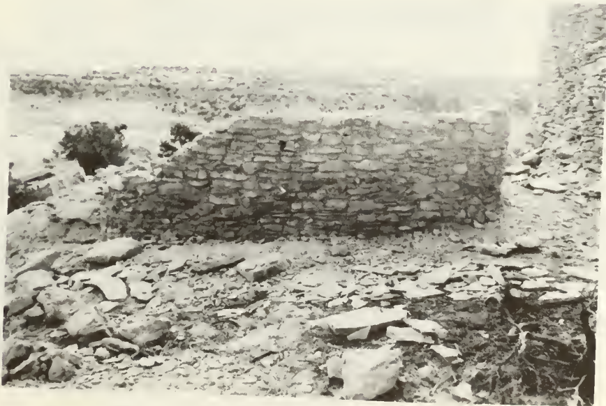
"After" stabilization; the west wall of room 4. (looking east)
