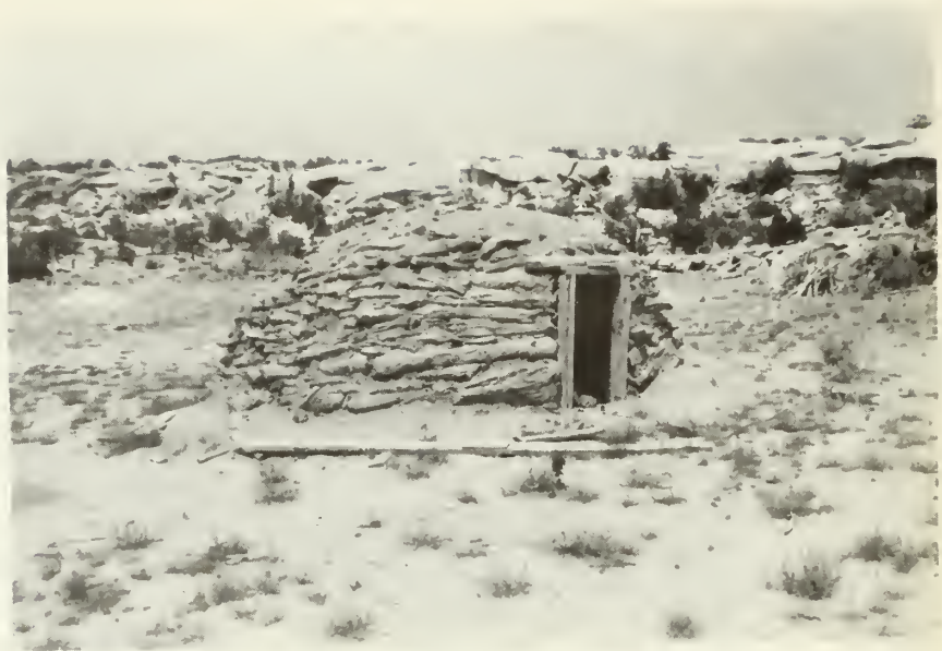
CM-186. Recent winter hogan built in the cribbed-log style. Note the lumbered wood used in the door frame. (looking west)
