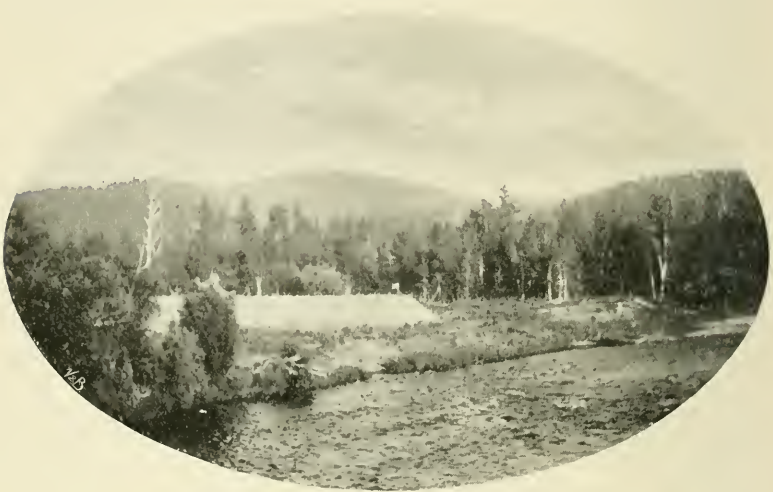
A break in the embankment in Trans-Baikalia.
