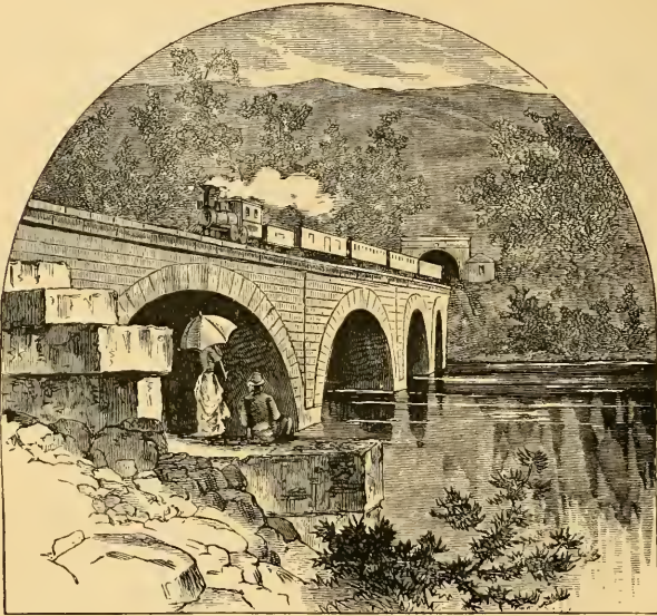
TUNNEL AT PHENIXVILLE, PA.
