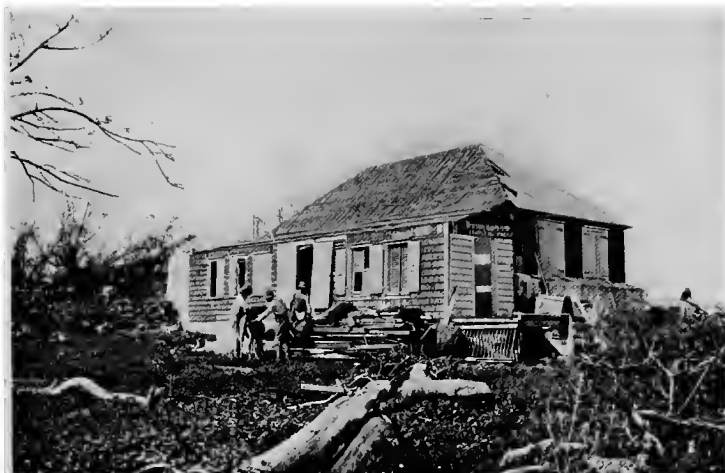
CANAAN ESTATE HOUSE, AFTER HURRICANE
