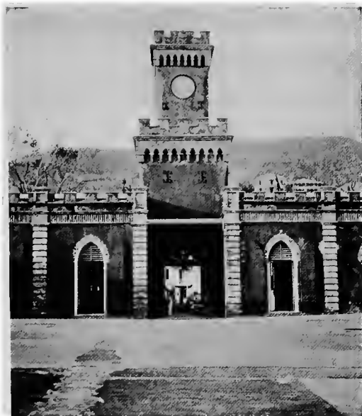
FRONT ENTRANCE OF CHRISTIAN'S FORT FROM COURTYARD INSIDE
