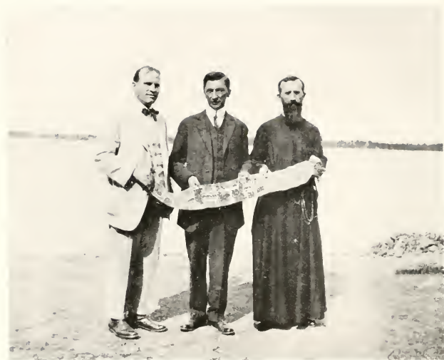
On the banks of the St. Lawrence at Caughnawaga, Quebec.
