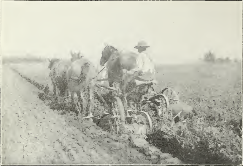
FIG. 1.—PREPARING LAND FOR SUGAR BEETS BY PLOWING UNDER A CROP OF ALFALFA, ONE OF THE BEST GREEN FERTILIZERS WHEN THUS TREATED IN THE FALL.
