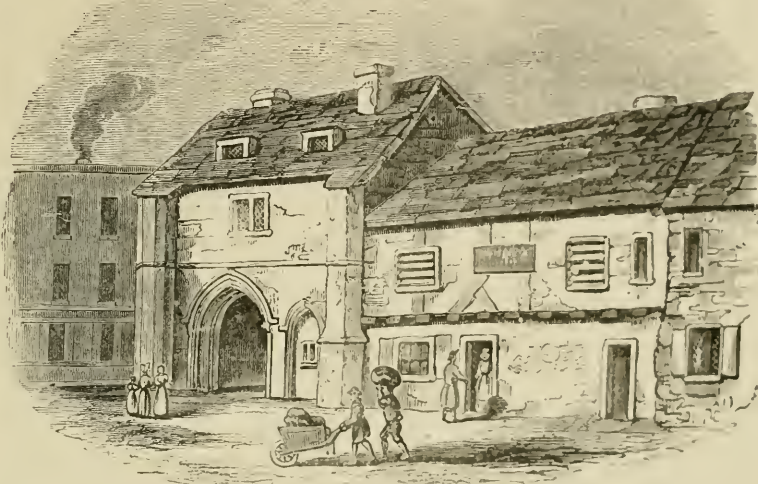
Bermondsey.—Remains of the Conventual Buildings.
