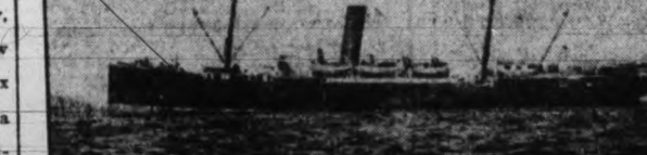
Forty years ago the Union Steamship Company of New Zealand placed its first transpacific liner, the Mararou, in service. She was the first triple expansion steamer to run on the Pacific, and so well-faithfully was she built in hull and engineering that she was converted into an oil-burner.
