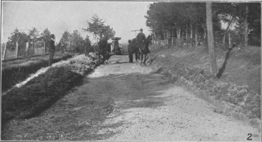
FIG. 2.—SUBGRADE READY FOR MACADAMIZING.
