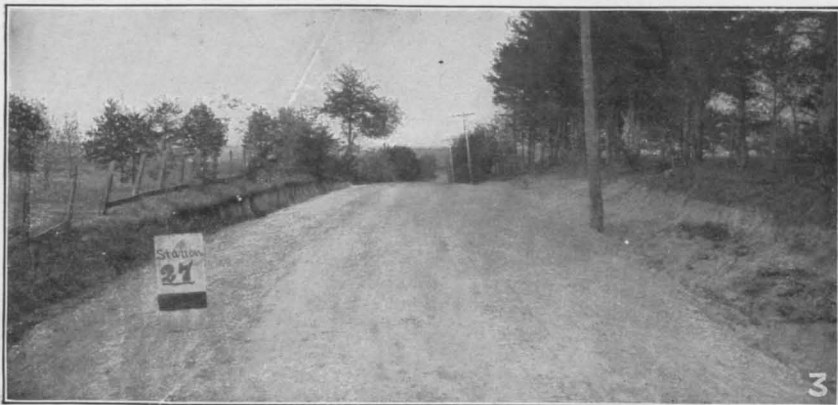
FIG. 3.—FINISHED MACADAM ROAD.
