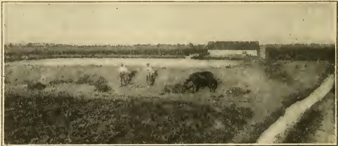
An earth reservoir used for storing water for irrigation. To the right is a main ditch leading to the field.
