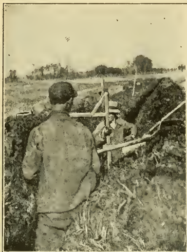
Digging a drainage ditch.
