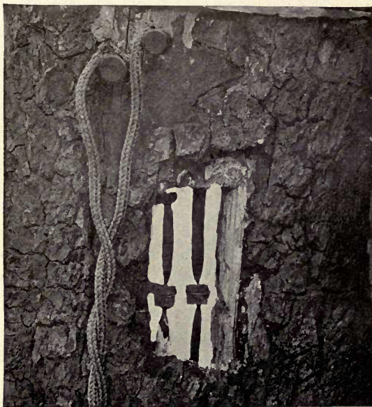
SECTION REMOVED SHOWING MICROPHONE
